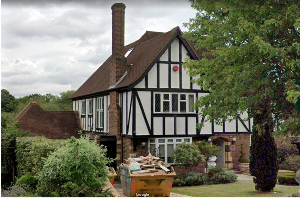
Figure 2. Front Elevation 1 (Copyright© 2021 Google)
