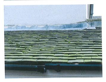
Some of the plain tiles are raised because they are warped. These were checked with an endoscope and they do not lead to other areas of potential bat roosting. One tile is lifted sufficient for bats to crawl under. It does not lead to other areas for bat roosting.
