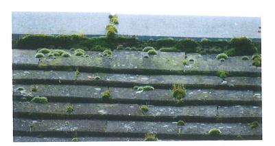
There are a number of missing plain tiles on the roof of the two storey part of the dwelling. These give access to the space between the rear of the plain tiles and the roofing membrane. There is no access to roof space and the underfelt could only be checked at the eaves where it was revealed to be a brittle bitumous underfelt of tar paper. There is access in a n umber of places but this area will not be affected by the proposed extension.
