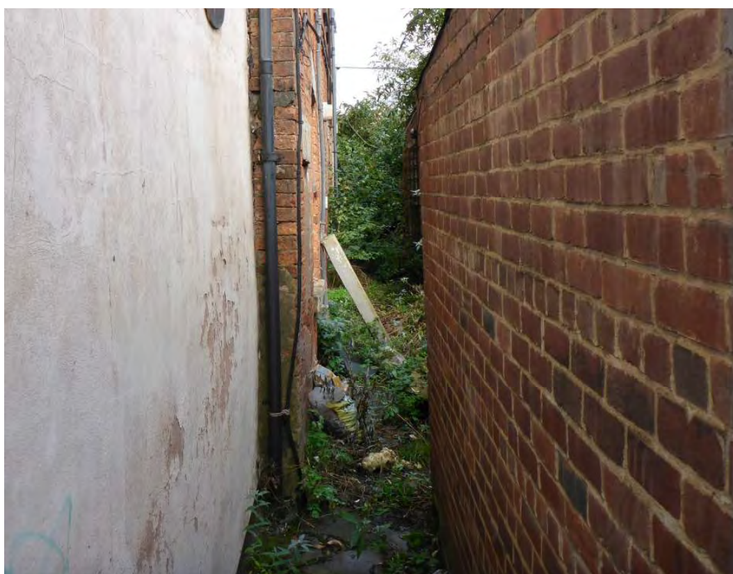
Plate 10: Site of covered passage leading to main yard
