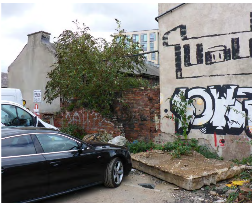
Plate 14: Rebuilt northern boundary wall
