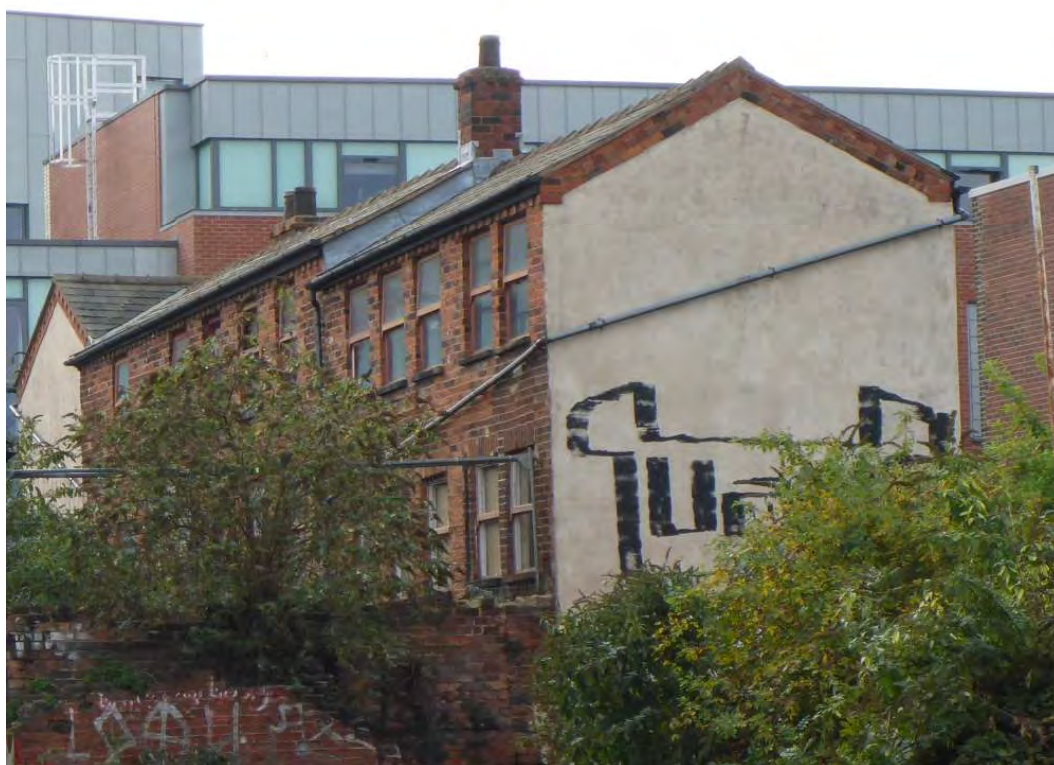
Plate 13: No.56, east elevation, looking south
