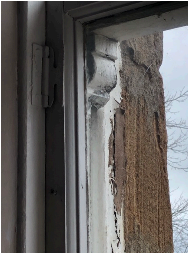
This is the original horn style to the building which we will take a template of and use in manufacturing new windows to retain the original design
