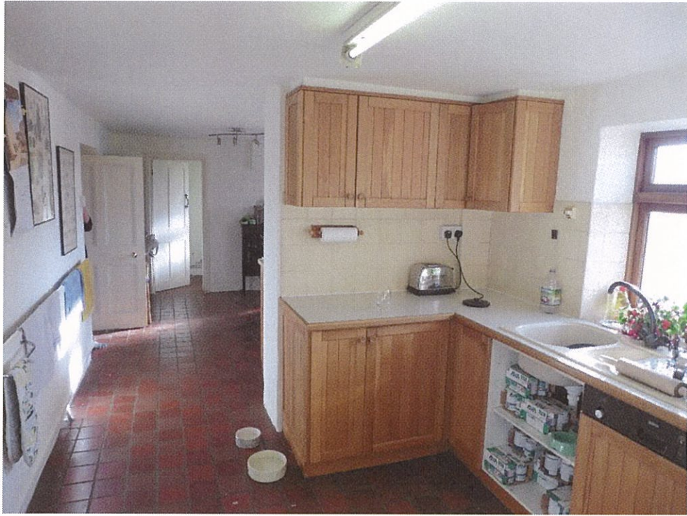
2. Wall in Kitchen to be removed
