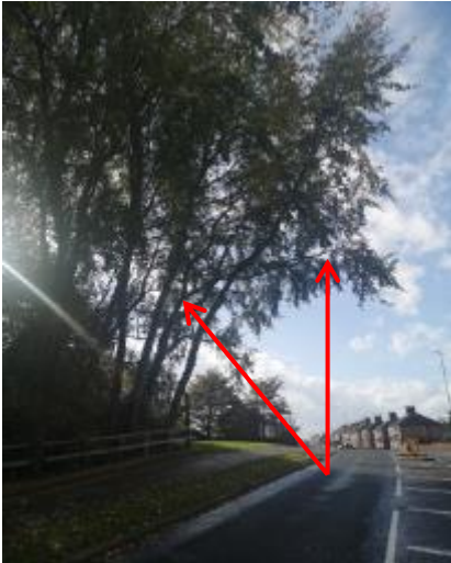
Figure 1: Leaning tree over main road G1 and over extended limb (arrowed).
