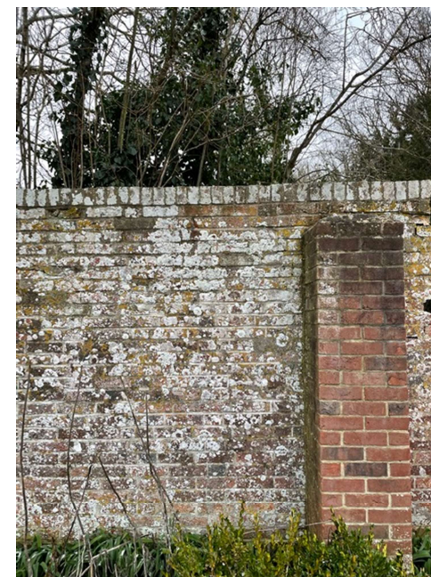
Image E – existing brick bond – Flemish Garden Wall bond & part site plan detailing location
