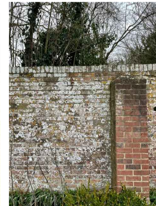
Existing wall - brickwork bond
