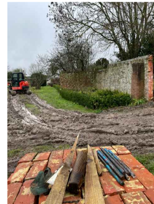
Existing wall - looking West
