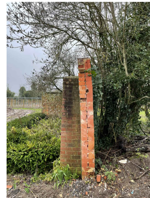
Existing wall - looking West
