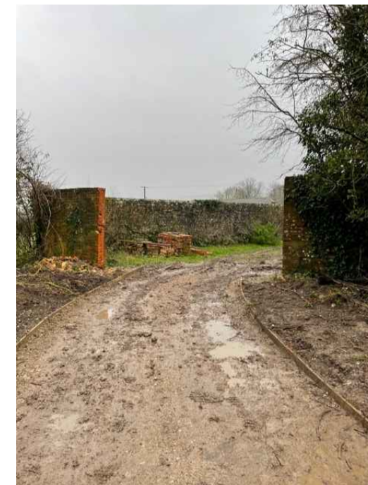
Existing wall - looking South
