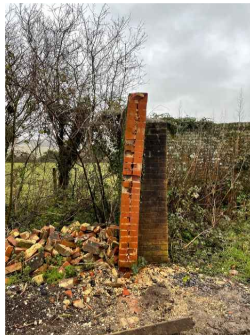
Existing wall - looking East
