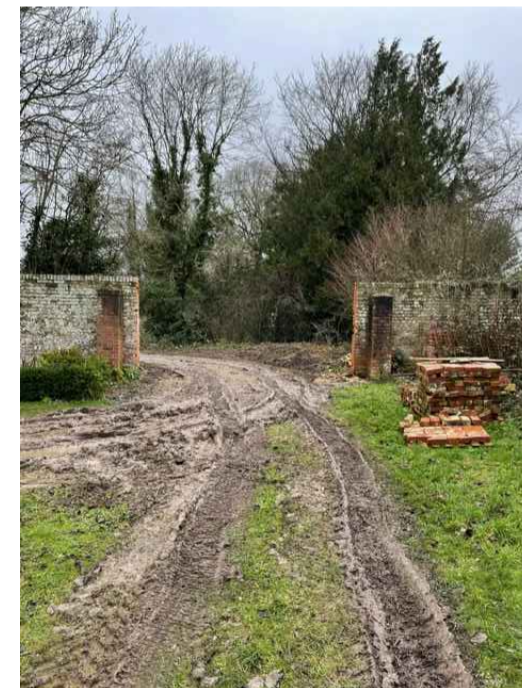
Existing wall - looking North
