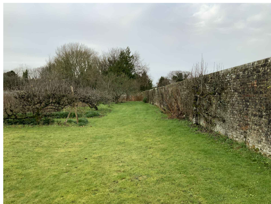
Existing wall - looking North
