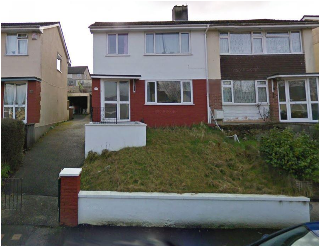
View of the front elevation
