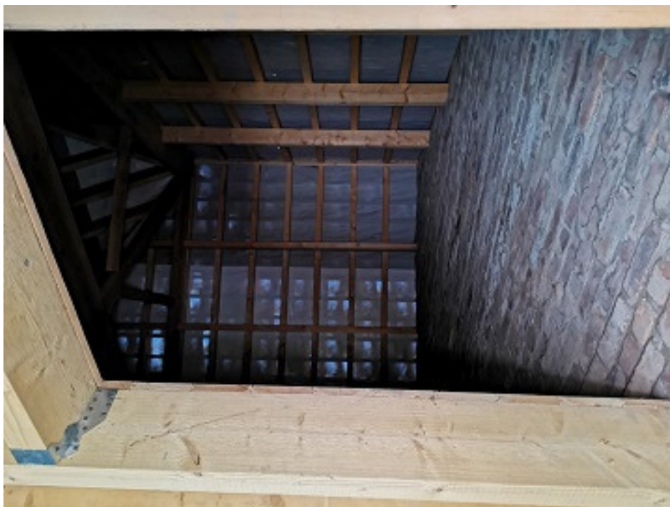
Plate 3. Shows the interior roof structure above the mezzanine floor
