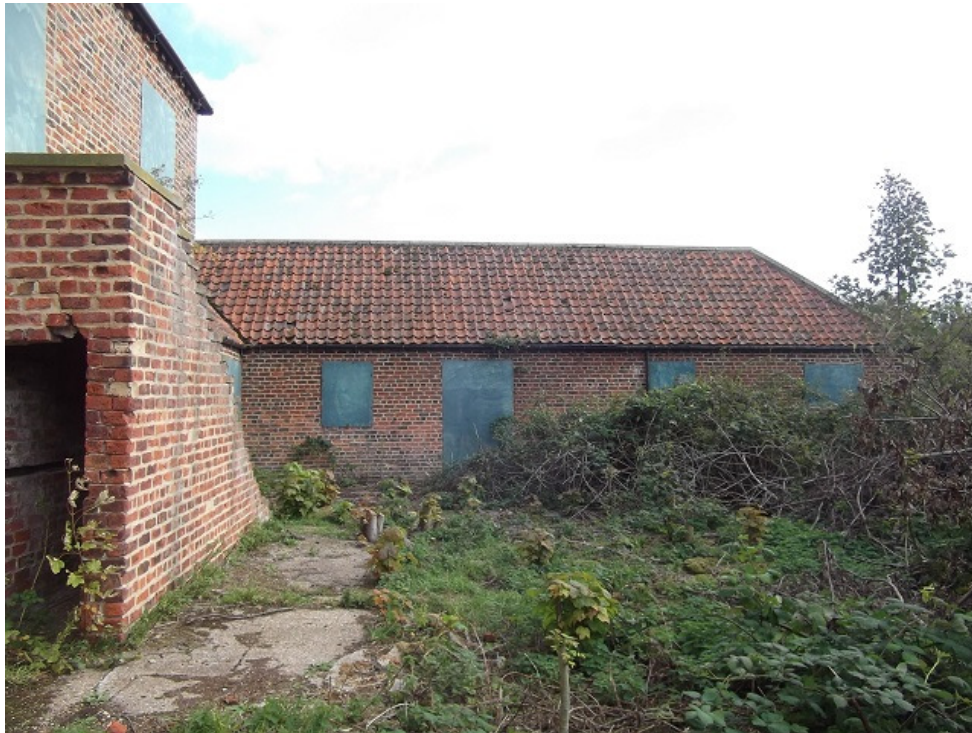
Plate 5. Looking towards the west elevation of Building 2.
