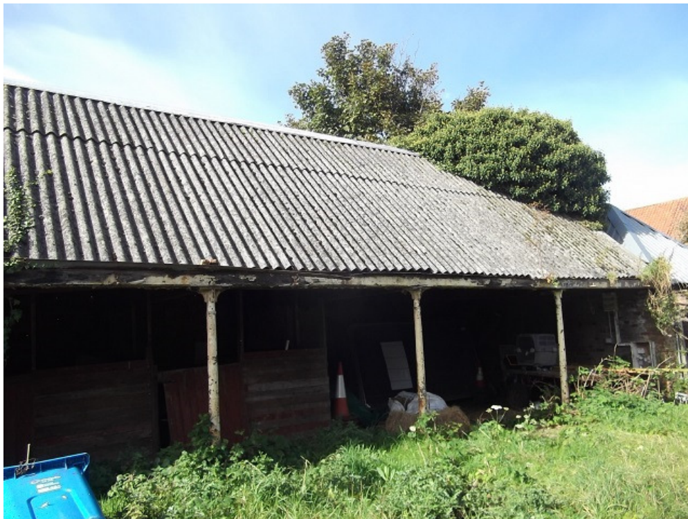
Plate 6. Shows east elevation of Building 3.
