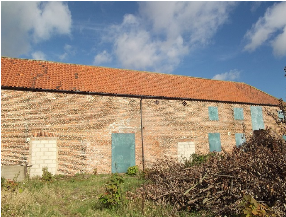
Plate 1. Looking towards the south elevation of Building 1.
