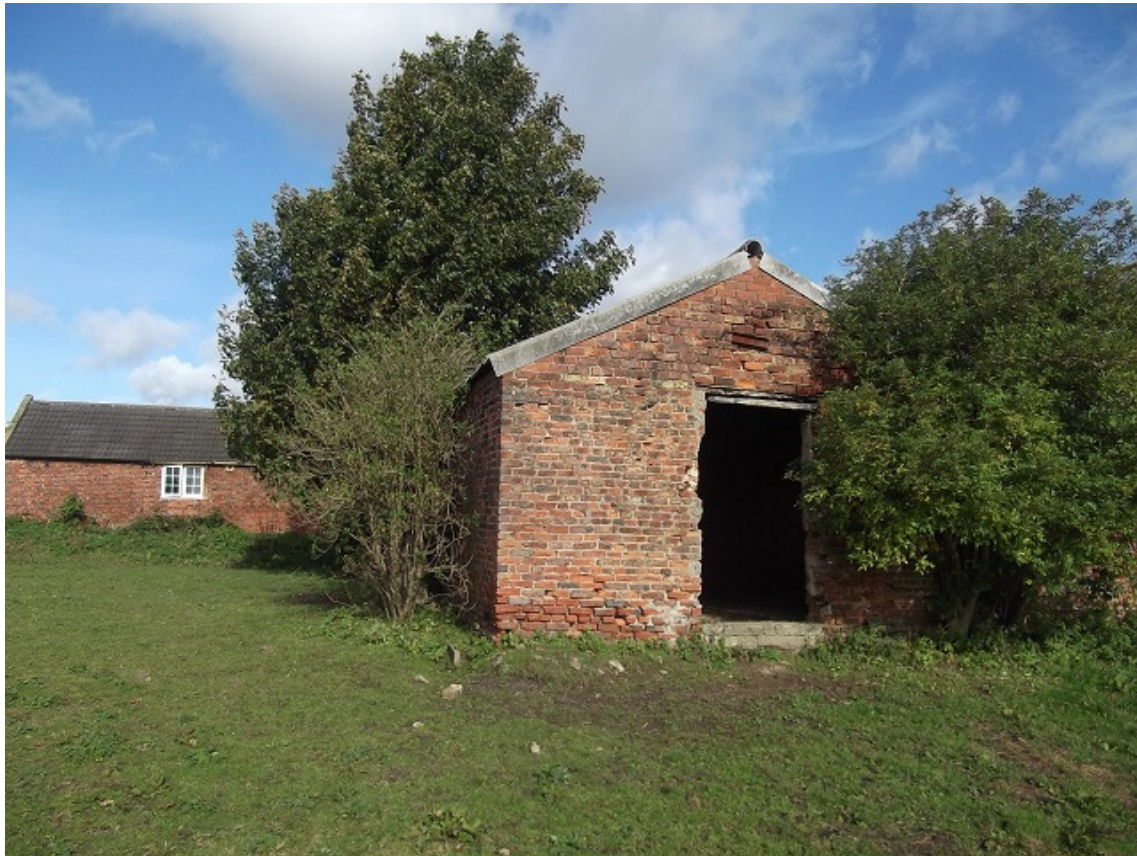
Plate 12. The south gable of the small outbuilding.
