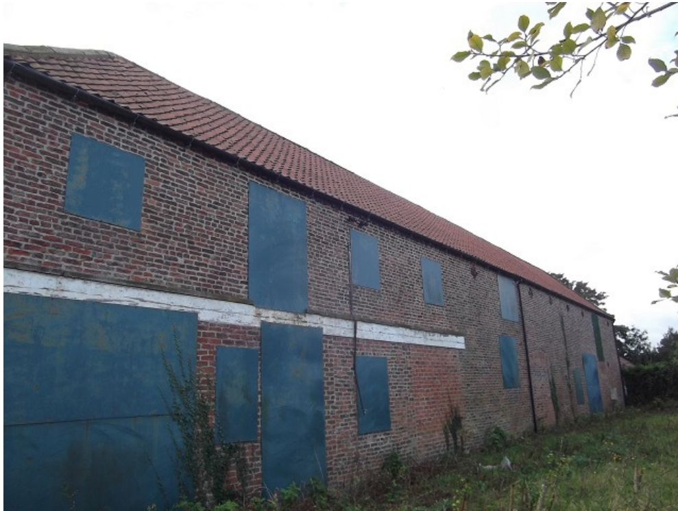
Plate 2. The north elevation of Building 1.
