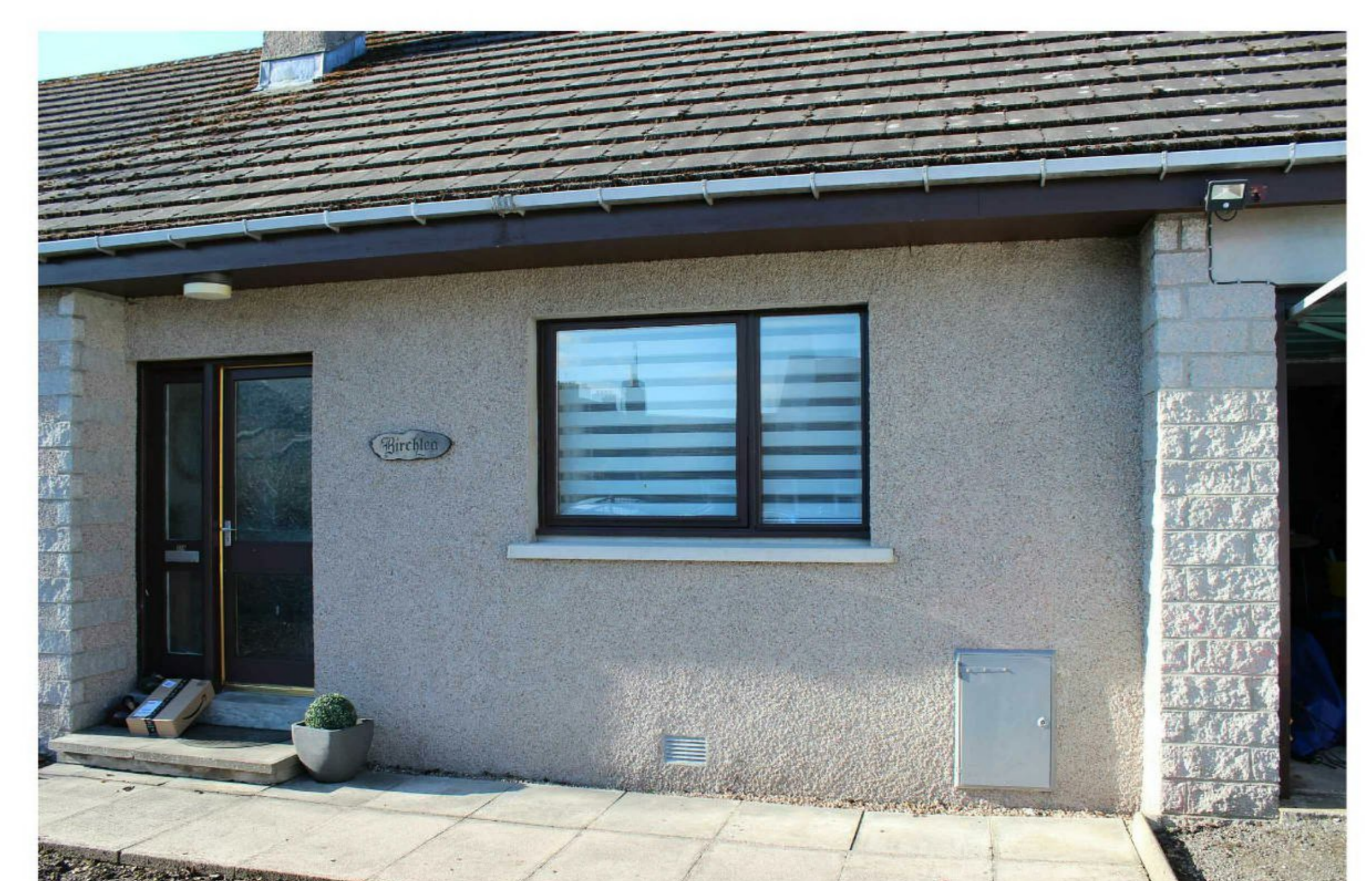
EAST ELEVATION FROM GARDEN WALL: Front Entrance Door & Bedroom Window.
