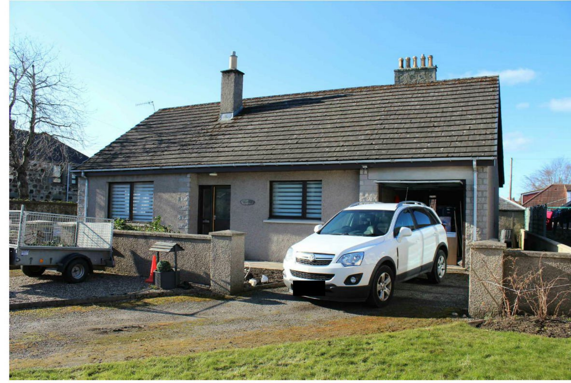
EAST ELEVATION FROM DRIVEWAY: Front Entrance Door, Lounge Window & Bedroom Window.
