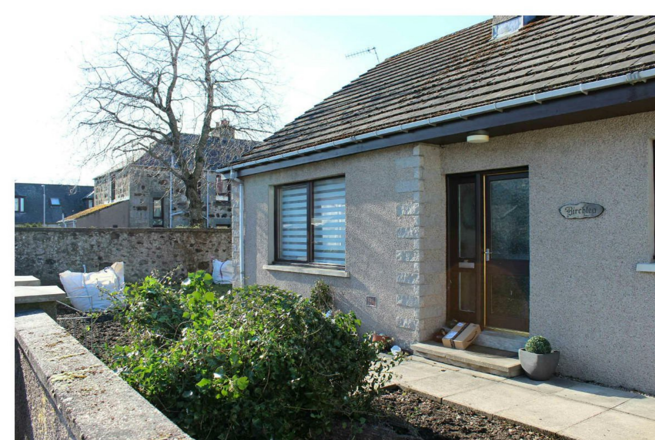
EAST ELEVATION FROM GARDEN WALL: Lounge Window & Front Entrance Door.
