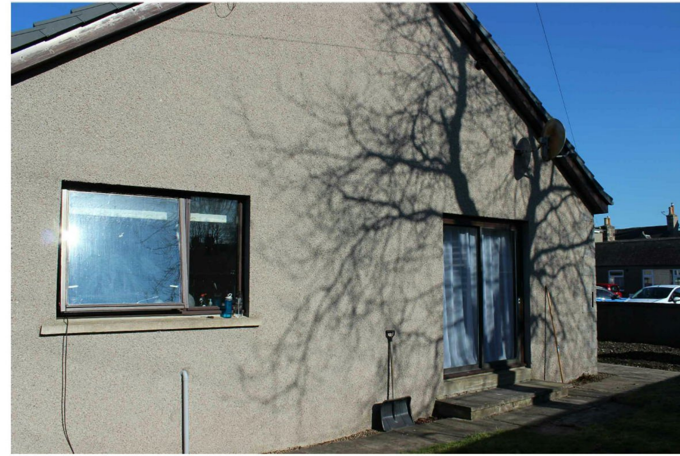
SOUTH ELEVATION FROM GARDEN: Kitchen Window & Lounge Sliding Door.
