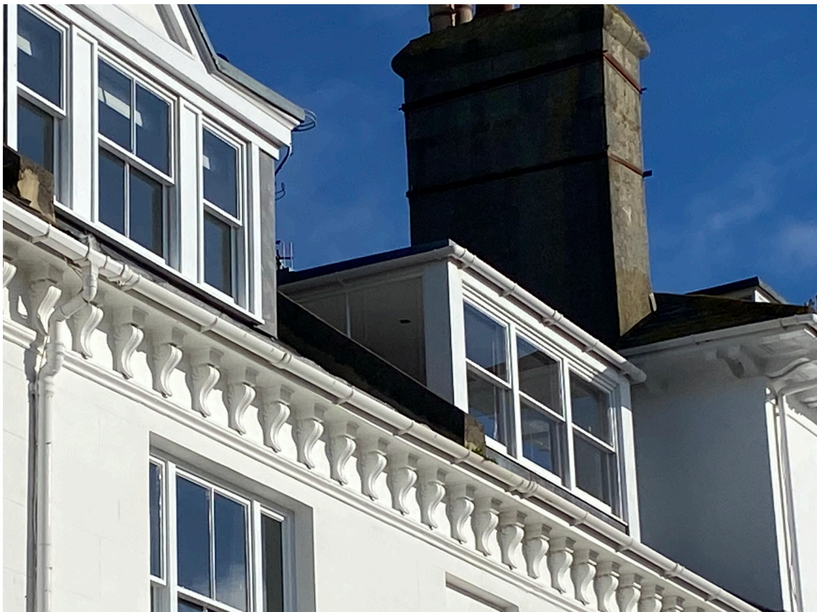
Photo 03. View of glazed flank elevation to dormer on Clifton Terrace.
