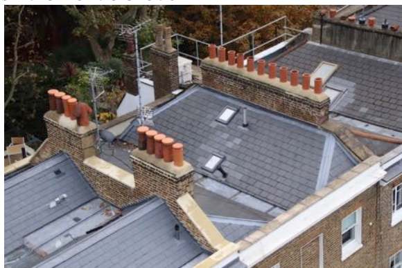
Photo 5: Upshot photograph of the right-hand side of roof.
