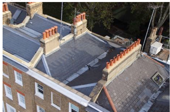
Photo 6: Upshot photograph of the left-hand side of roof.
