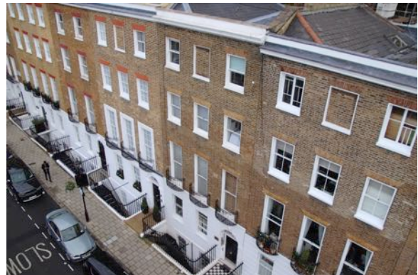
Photo 4: Upshot photograph of the front elevation.
