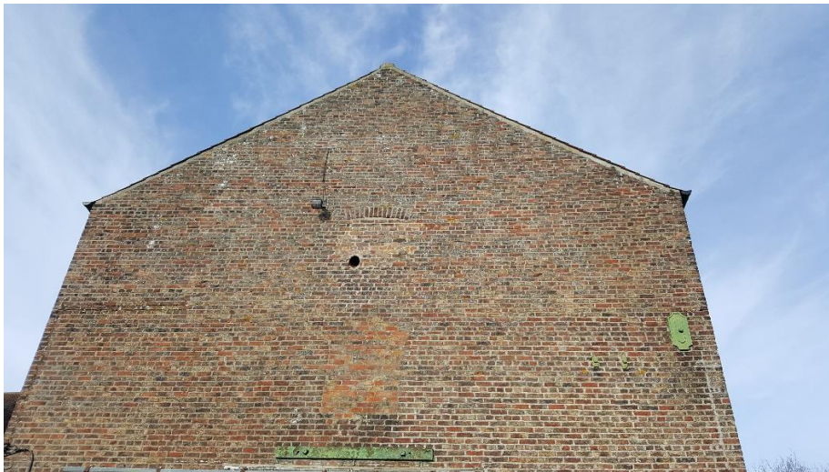
Plate 9: the southern gable end of the warehouse.
