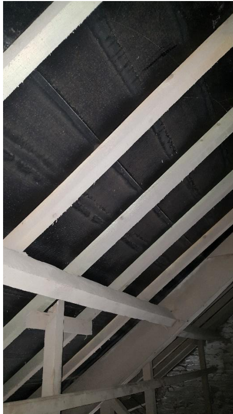
Plate 11: the interior roofing felt.
