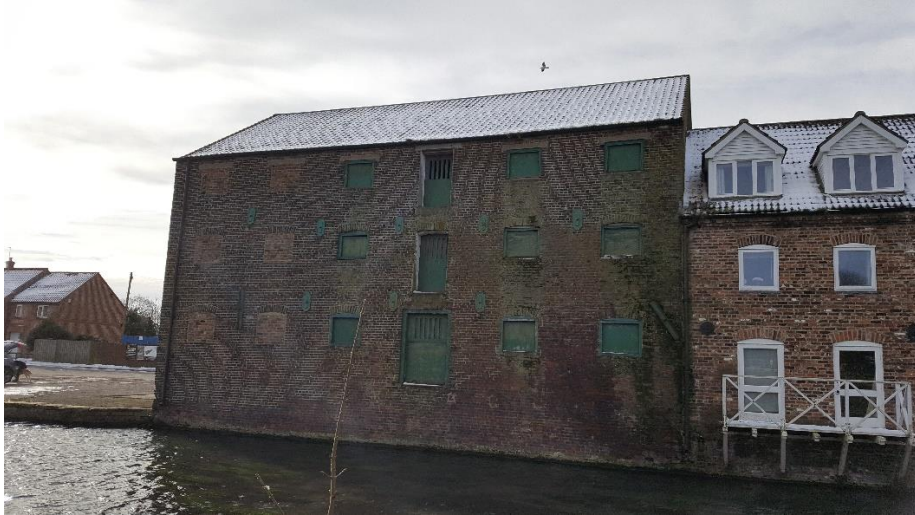
Plate 5: the doors and windows on the eastern aspect.
