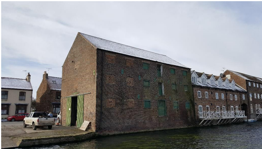
Plate 2: the warehouse is adjacent to the canal. Photograph taken from the south-east.
