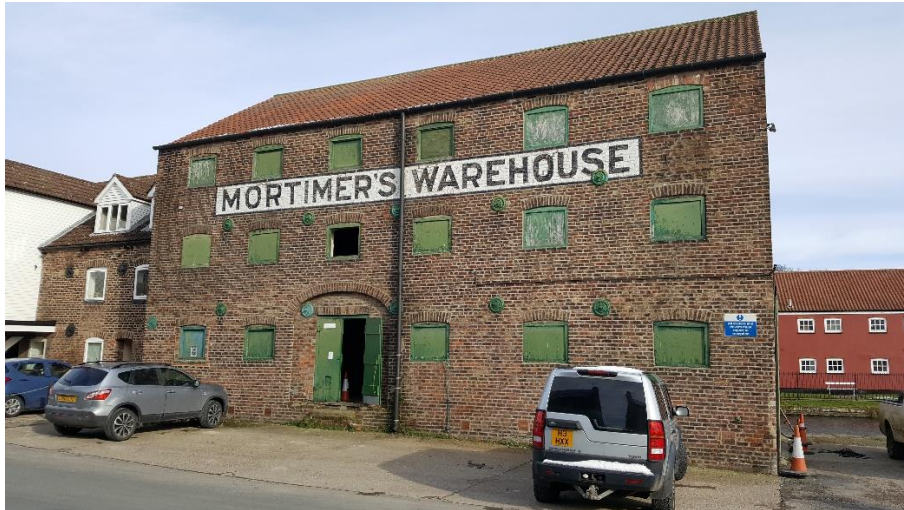
Plate 3: the door and windows on the western aspect of the warehouse.
