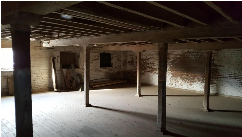
Plate 6: the northern part of the interior of the first floor.
