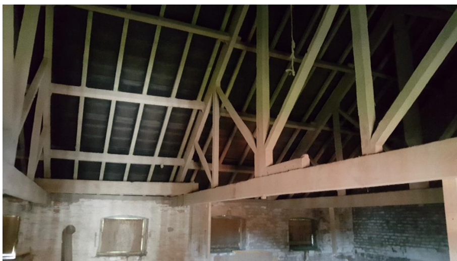
Plate 10: the interior timber frame of the roof.
