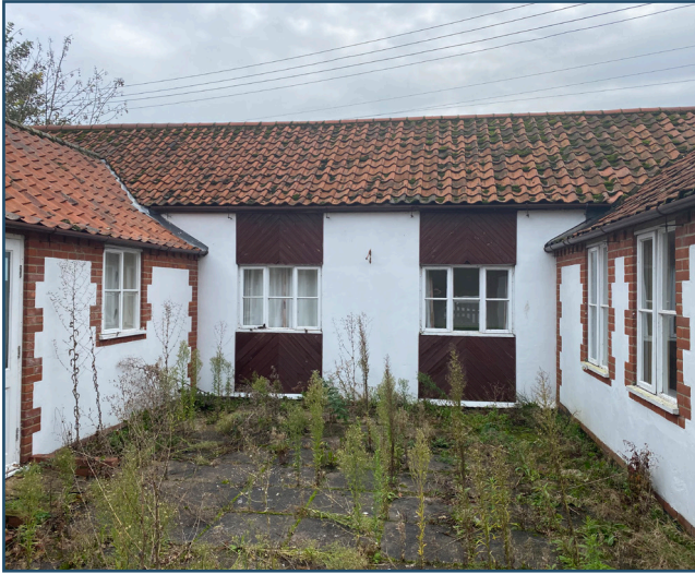
Existing building - West Courtyard Elevation
