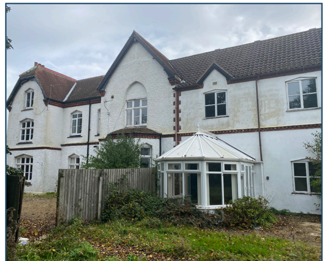
Existing building - East elevation
