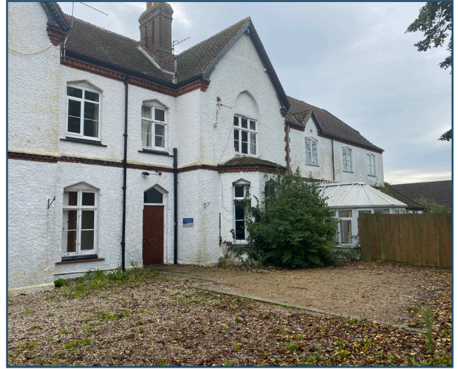
Existing building - Main Entrance
