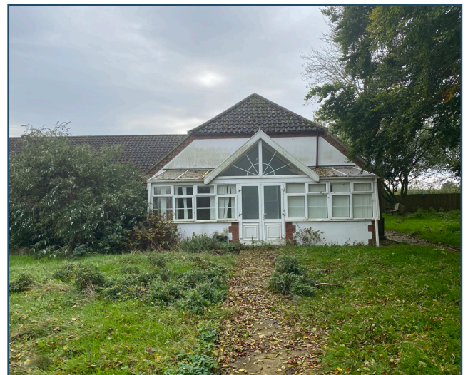
Existing building - West Entrance
