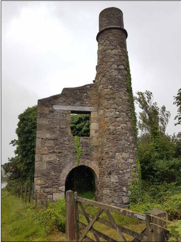
Plate 1: Eldons Engine House looking southeast from the highway
