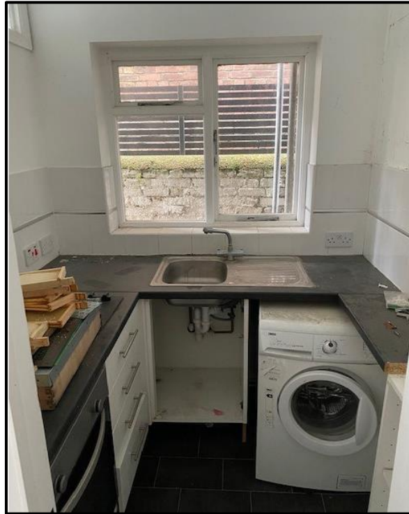
(Existing kitchen Flat 2)
