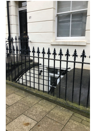
Railings to front lightwell
