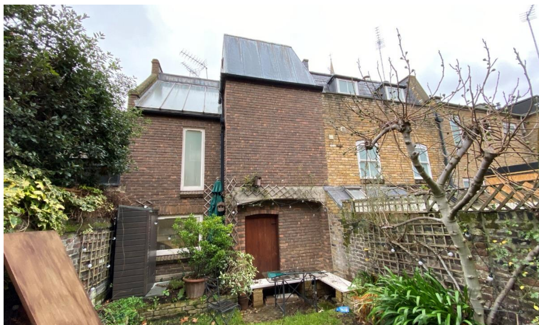
Figure 2 View of rear of application property
