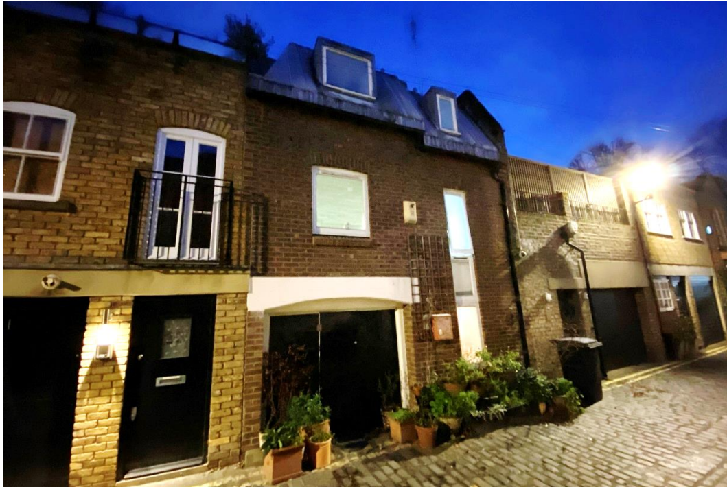
Figure 1 Photograph of the front of 25 St Petersburg Mews (as existing)
