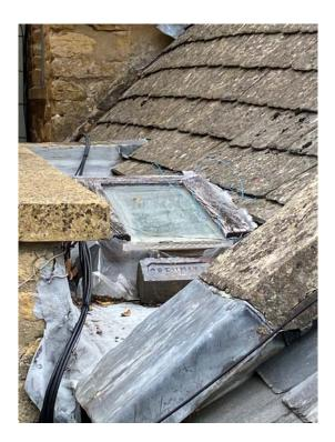
• Following remedial works to rooflight over Kitchen, replace flat roof covering with grp covering. Allow for inspection of lead flashings and include allowance for replacing 2 lin/m of flashings with Code 5 lead if required. Roof area 1.9m2
