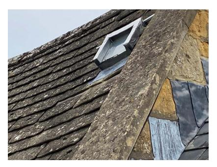
• Prior to replacement of flat roof covering, investigate leaks from flat roof light. Replace flashings where necessary. Repair damp staining and make good decoration internally
