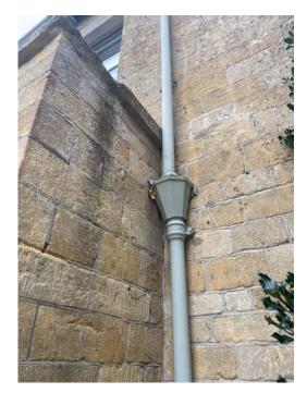
• Following works to the rainwater outlet, replace flat roof covering with grp covering. Allow for inspection of lead flashings and include allowance for replacing 3 lin/m of flashings with Code 5 lead if required. Roof area 1.9m2
