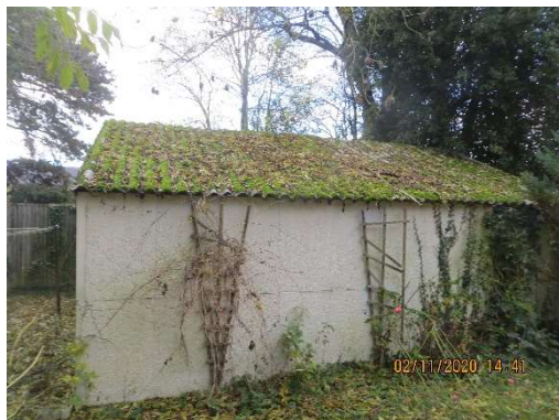
Photo 6 – garage / outbuilding to the rear of the site
