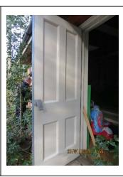
Solid timber panel door, painted, generally in good condition with single yale lock. Push button internally. Repair and redecorate
