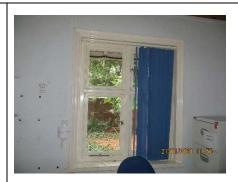
Timber casement windows with opening right casement and fixed casements to the left at low level. 1nr openable casement at high level. Single glazed with a concrete sill. Original ironmongery. Single pane of glass broken. Single glazed.
