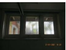
Single glazed Georgian wired timber casement window with 2nr fixed lights to the left and right and a central opening casement with original ironmongery, stay and catch and locking mechanism.
