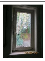
Timber single glazed casement window with original ironmongery. No locking mechanism with a concrete sill.
