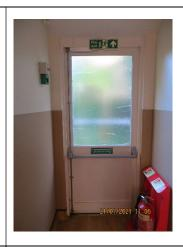
Timber door with glazed top light and fixed panel at low level. Toughened glazed unit with timber frame and push bar on the inside. Frosted assumed toughened.
