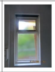
Timber glazed casement window with opening top light fixed to bottom light.
