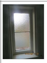
Stippled glass, single glazed metal crittall casement set into a timber frame. Window stay and catch original, unlikely to operate. Single glazed.
