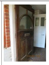
Hardwood panelled door with single pane glazing at high level. Frosted central panel and stippled glass above with letterbox, brass doorknob, yale lock and high level handle along with magnetic catch.
