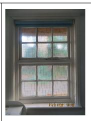
Timber casement with opening light top hung with a fixed lower casement with integral timber beading and Georgian wired glass. Original stay for top hung casement. Concrete windowsill. Georgian wired.
