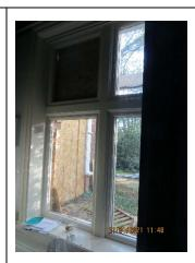
Timber single glazed Georgian wired window set into a concrete frame with a concrete sill. All fixed casements. Georgian wired.
