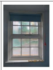
Timber casement with opening light top hung with a fixed lower casement with timber beading and Georgian wired glass. Original stay for top hung casement. Concrete windowsill.
