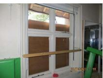
Timber casement windows with opening right casement and fixed casements to the left at low level. 1nr openable casement at high level. Single glazed with a concrete sill. Original ironmongery. Single glazed.
