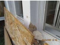
Large ground floor bay to the rear of the property. Metal crittall casement windows at low level. Opening low level casements to the right and left of the bay with 2nr fixed casements centrally and to the angled sections. Leaded metal crittall casements at high level with a single opening casement centrally. All with original ironmongery. Casements set within a concrete frame which requires repair following fixing of hoarding along with a concrete sill. Timber frame internally. Single glazed.
