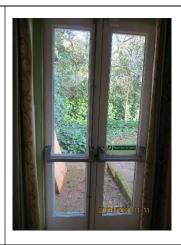
Double door set with glazed top and bottom lights and drip bar at low level along with fire escape ironmongery internally and toughened slimline glazed unit. Repair and redecorate. Fire ironmongery to be checked for compliance.
