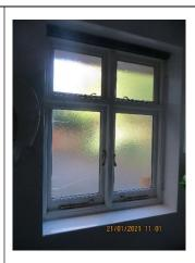
Timber casement window with opening top and bottom casements. Toughened glazed units with a frosted glass and a concrete sill. Frosted assumed toughened.
