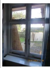
Timber casement window with opening top and bottom casements. Toughened glazed units with a frosted glass and a concrete sill.
