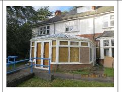
UPVC conservatory double glazed units with a number of blown and broken window and roof lights. Double glazed units assumed not toughened.
