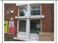
Metal crittall casement window set into a timber frame with 1nr opening light at low level and metal crittall casements at high level with leaded lights. All original ironmongery. 1nr casement has secondary glazing internally at low level. 1nr glazed unit has been replaced with toughened glass, the other is single glazed.
