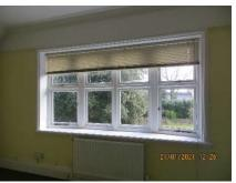
Large bay window at the rear which is a timber casement single glazed window with opening lights at the side and fixed casements. Windowsill is decayed along with casements where repairs are required.
