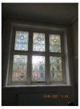
Stained glass window above front entrance. Timber fixed casement windows with 1nr openable window at low level centrally. Set within a timber frame. Original ironmongery.
