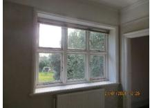
Window above the conservatory. Again, single glazed window with opening lights on the side and fixed casements. Appears that a film may have been applied to this window, but this cannot be confirmed. Sill again looks decayed.
