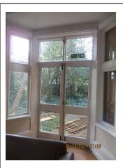
Timber glazed windows with Georgian wired glazing on the side lights which is window 32 and window 33. All set within a concrete bay frame. Twist handle to open internally with locking catches at low and high level along with magnetic catch strips. No opening lights. Window 32 & 33 is Georgian Wired. Door 34 is toughened.
