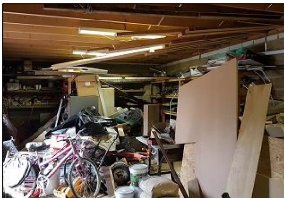
Figure 4: Internal view – first floor.
