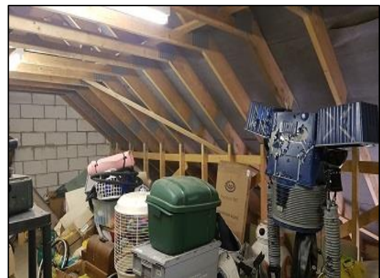
Figure 6: Second floor open to roof structure.
