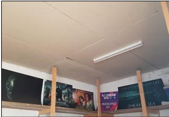
Figure 6: Northern aspect room with boarded ceiling.
