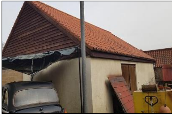
Figure 1: South and western aspects
