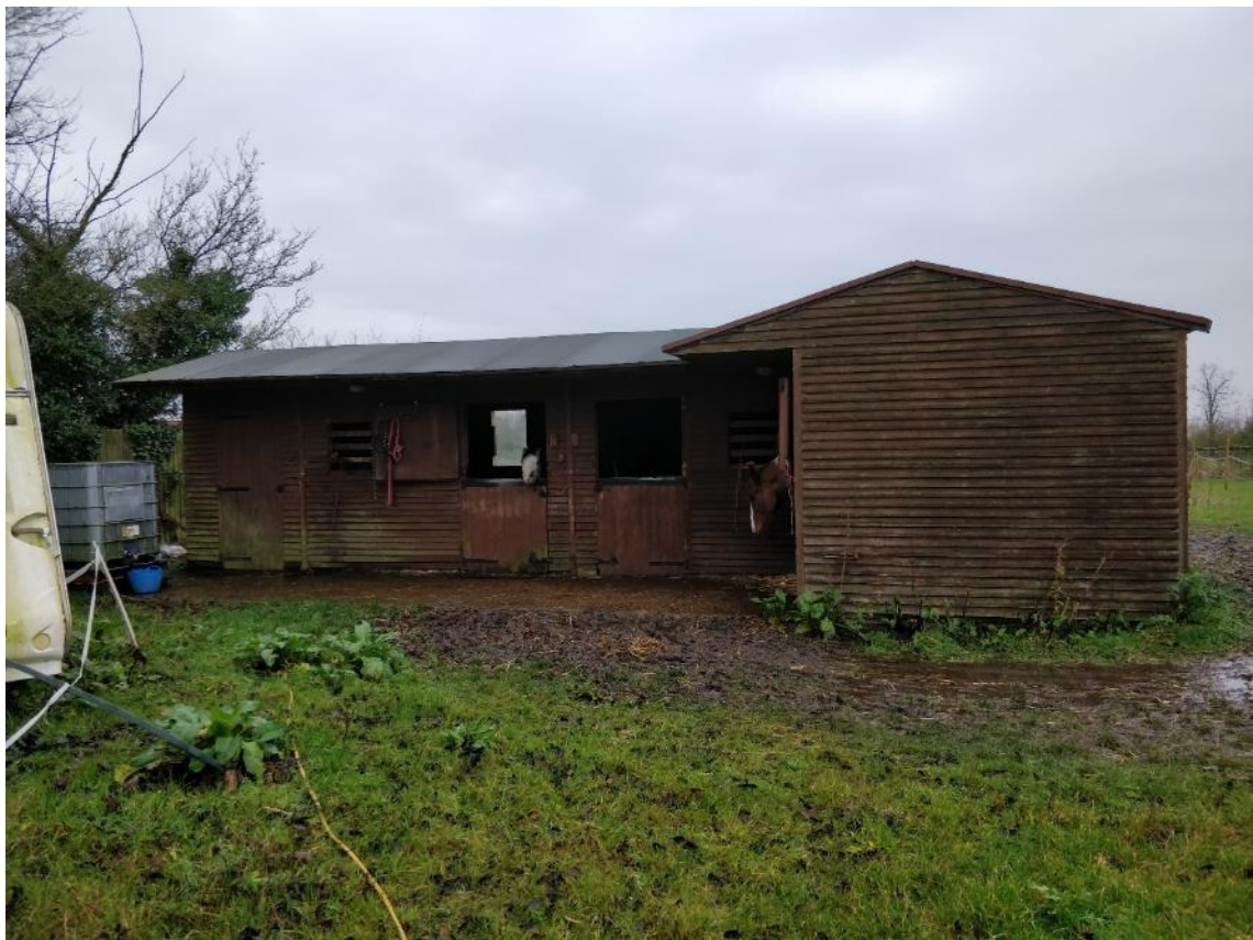
Photo 7 , east aspect of building one, looking west.
