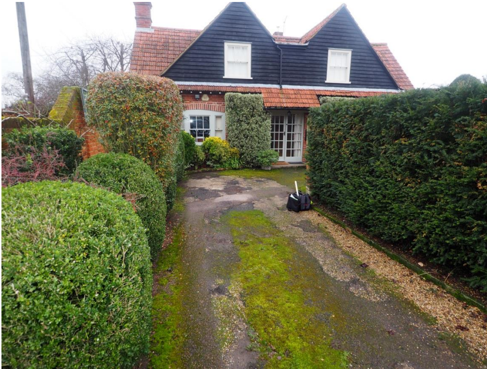
Figure 1: From the driveway looking east towards The Coach House.
