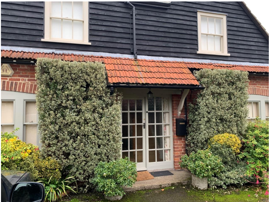
Figure 6: Looking east towards The Coach House's existing front door and Canopy.
