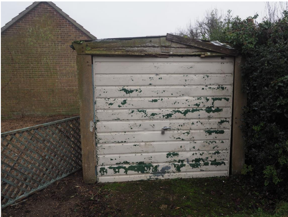
Figure 2: From Church Lane looking east towards existing garage.
