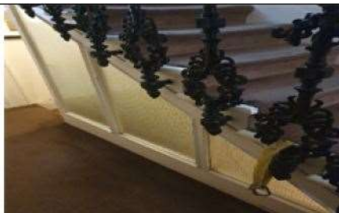
3. Basement partition to 45 Warwick Avenue
