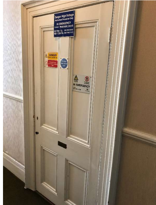
2. Ground floor intake door
