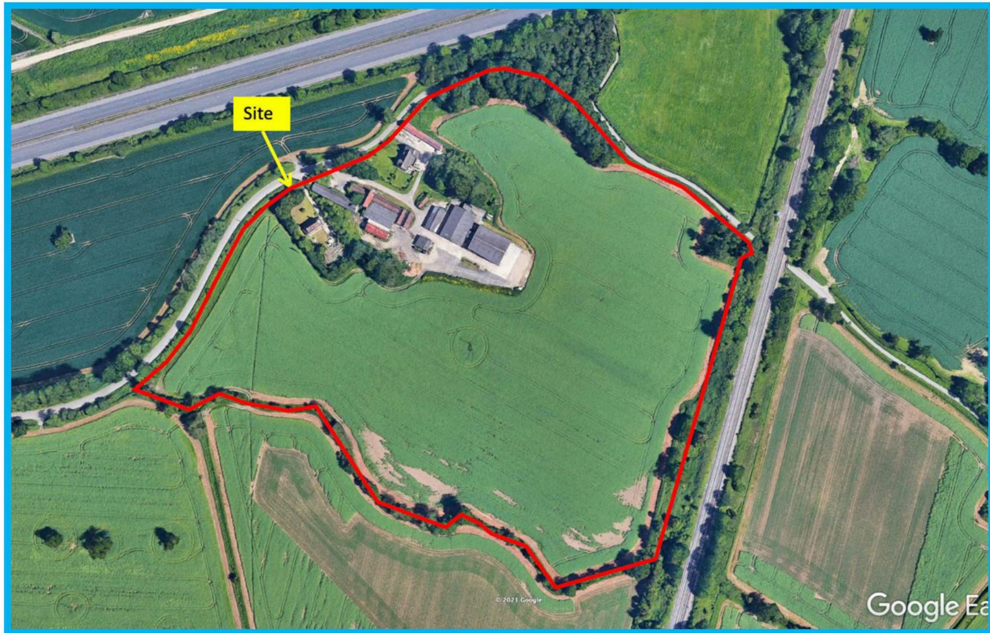
Fig 3 Satellite view of site (Google Earth).
