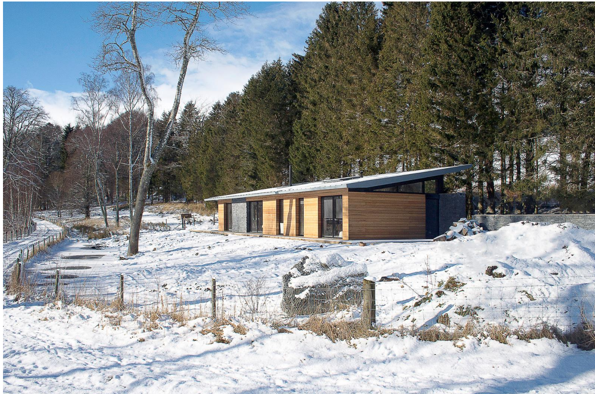
Fig.24 Strathdon House – Brown & Brown Architects
