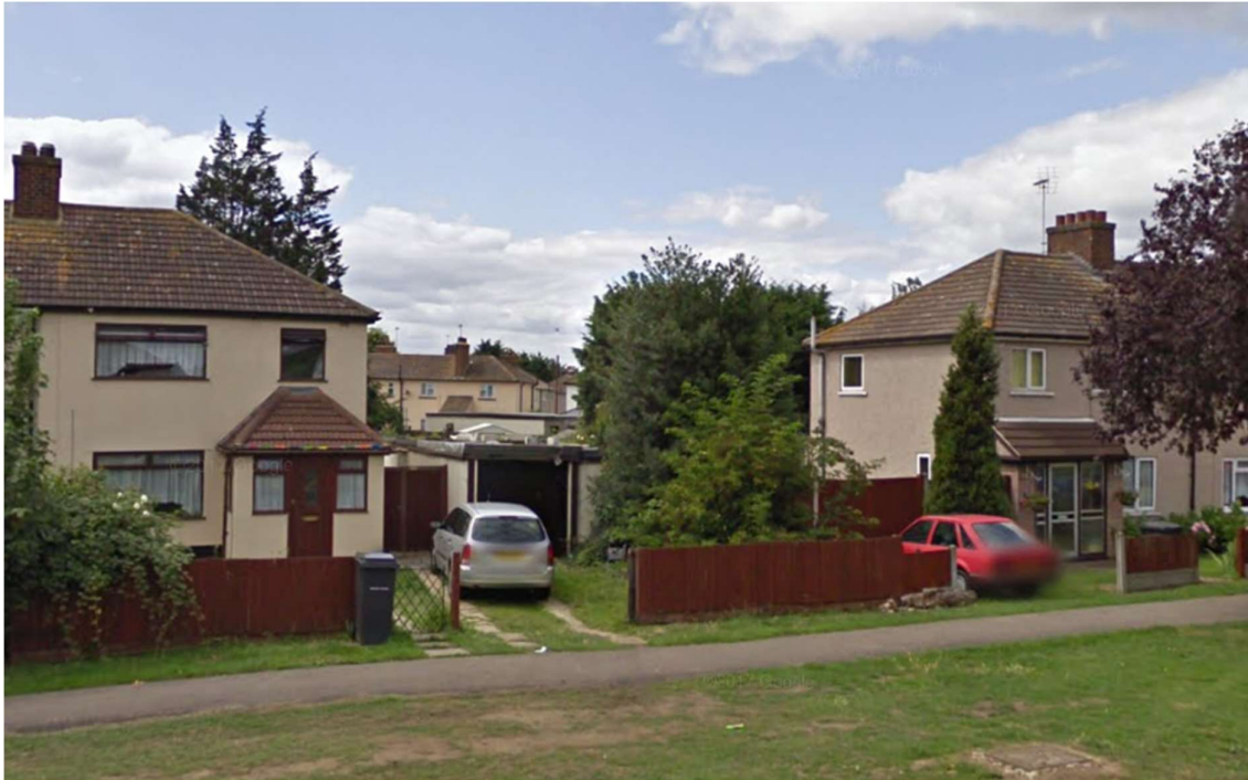
99-101 Feenan Highway - Front elevation dated April 2015 (Google Earth)
