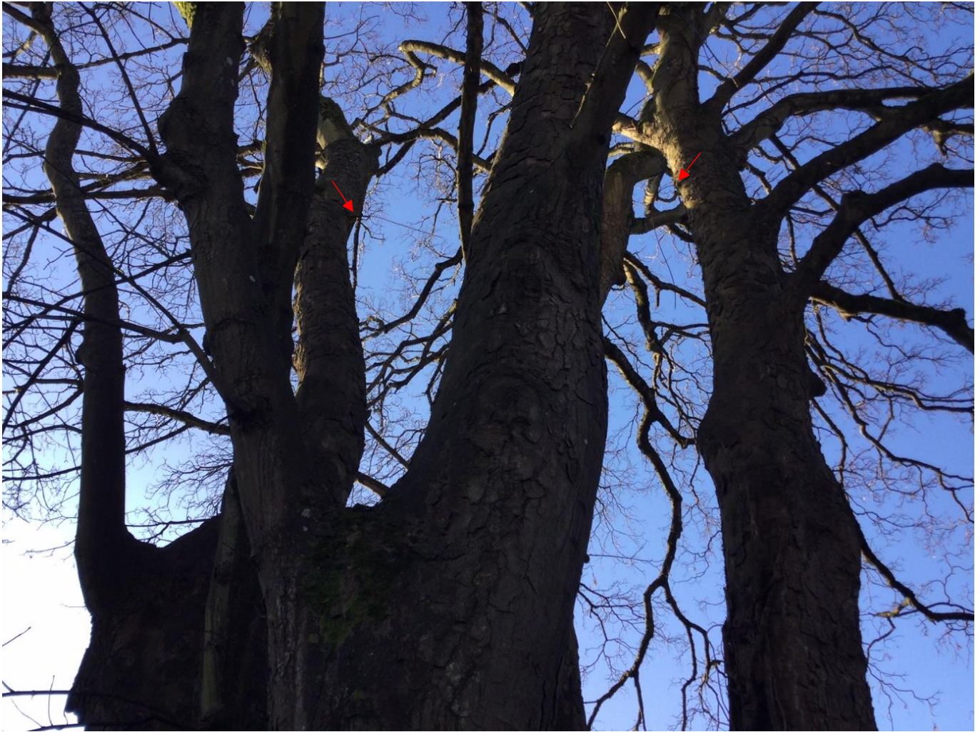
SAL5 T1 sycamore with failed metal cable bracing identified by red arrows.
