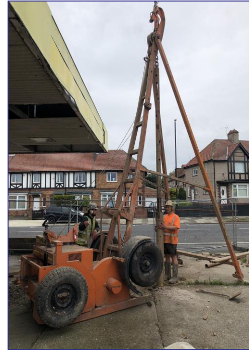
Photographic Plate 14 – CP1 being sunk.
