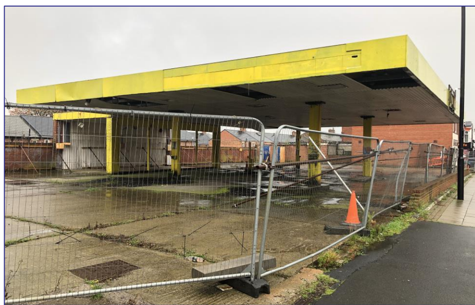
Photographic Plate 1 – The site, derelict petrol filling station.
