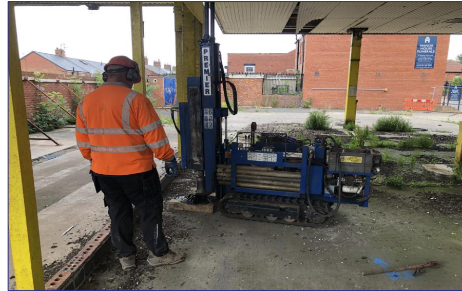
Photographic Plate 6 – WS5 being sunk in vicinity of former petrol pump islands.
