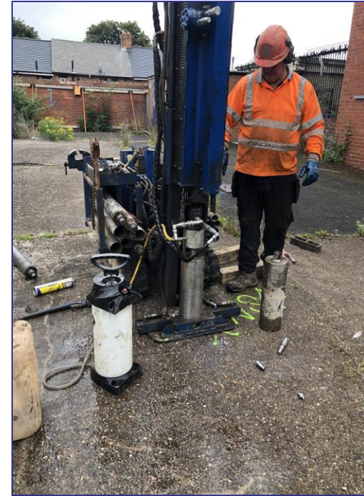
Photographic Plate 8 – Drilling rig coring through concrete for borehole WS4.
