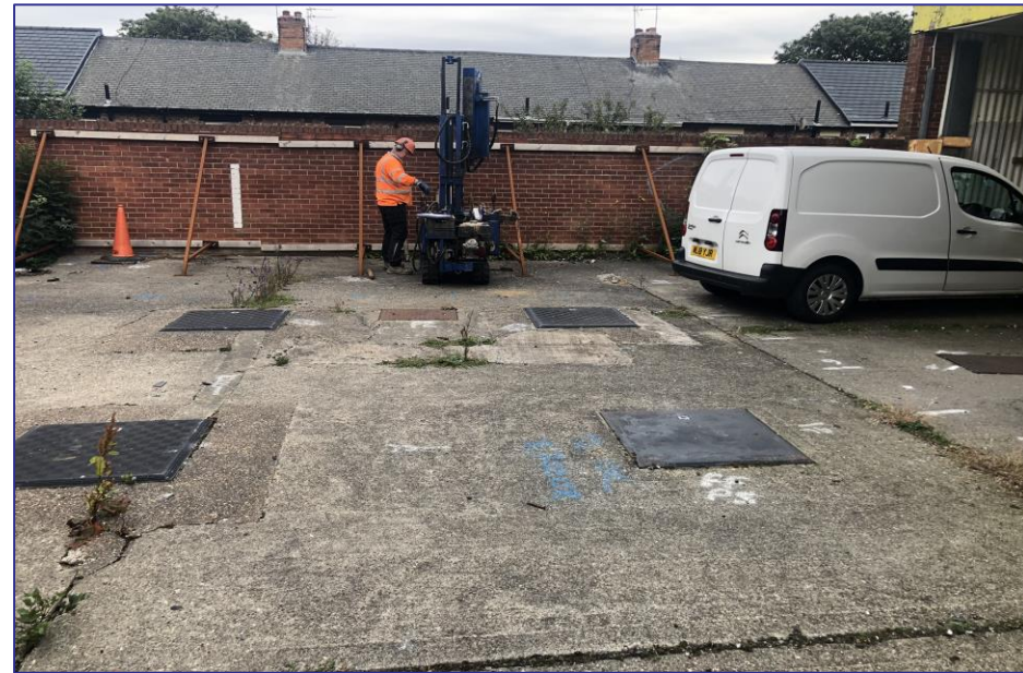
Photographic Plate 4 – Borehole WS1 being sunk.
