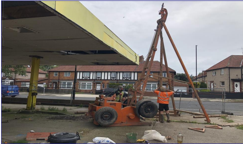
Photographic Plate 13 – Cable percussion drilling rig being set up on borehole CP1.
