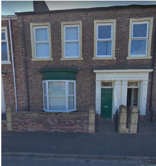
Photograph 1 – Existing Highway Elevation.
