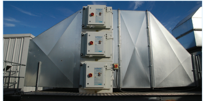
3 ESP Units Stacked in modular formation
