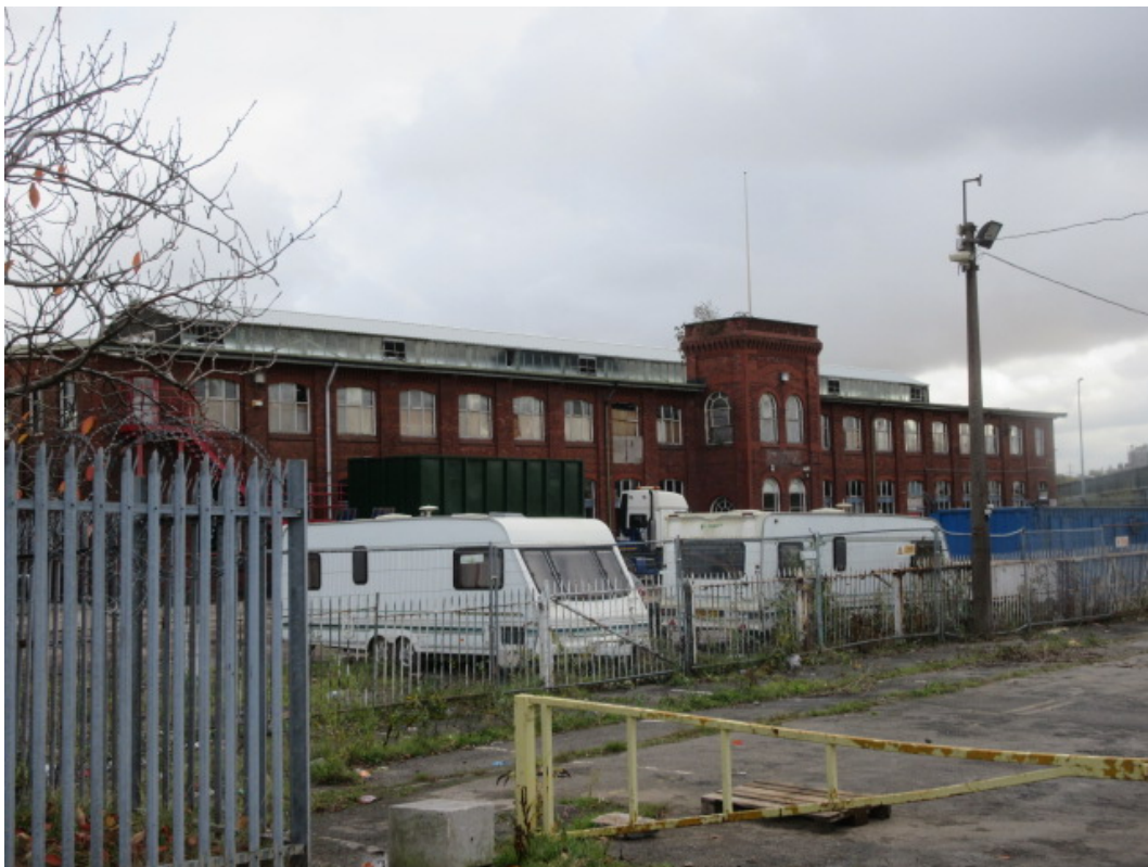
Plate 4: Southern site building, looking south east
