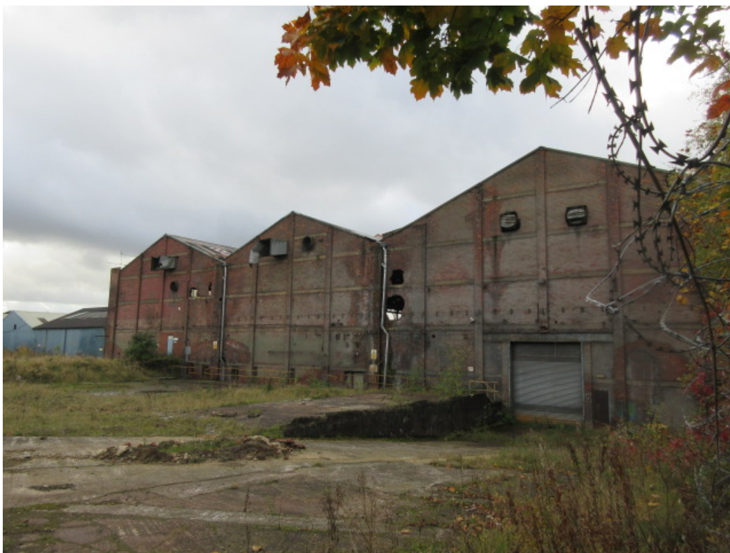
Plate 8: Rear of site buildings
