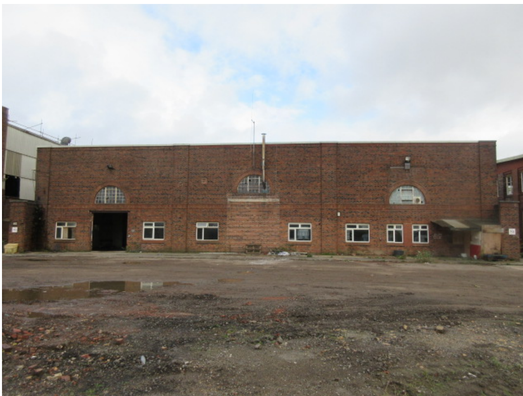
Plate 6: Central block, looking east
