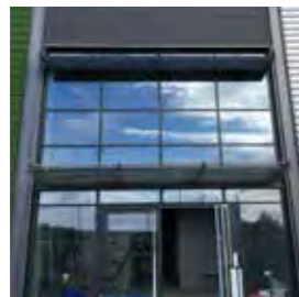
Main entrance Thermally broken Curtain Wall System with powder-coated aluminium frames
