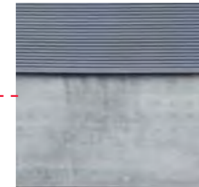
Precast Concrete Wall
