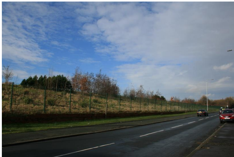
Figure 5. View looking Northwest towards G78
