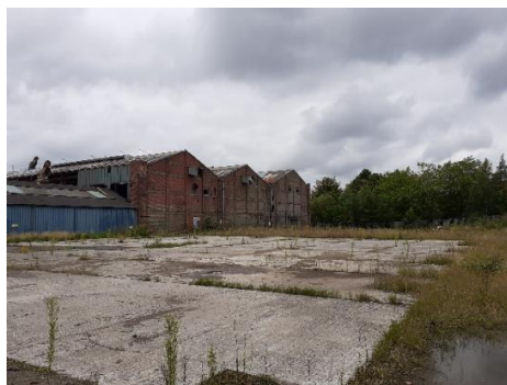
Figure 6: Hardstanding surrounding buildings within centre of site.
