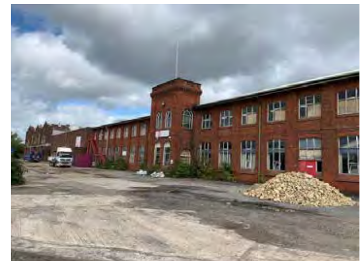
4. Looking north to existing foundry office building now dilapidated
