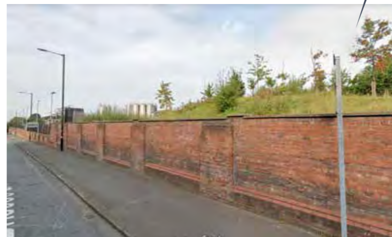
7. Boundary with Briscoe Lane, looking South West
