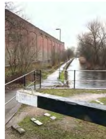
7. Looking south along existing warehouse
