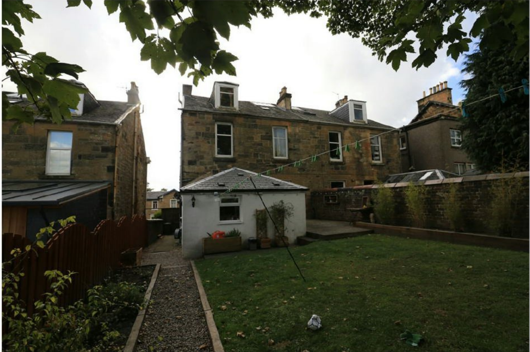
Next door extension roof
