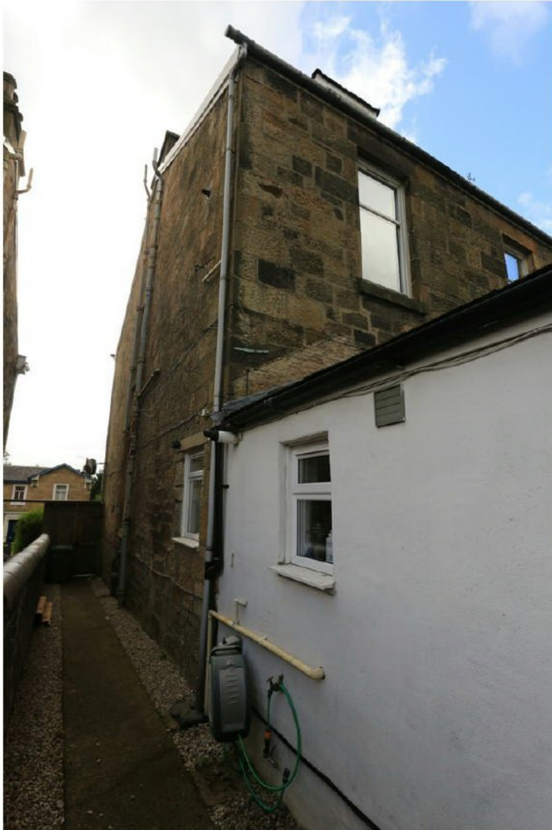
Existing side elevation showing white UPVC windows
