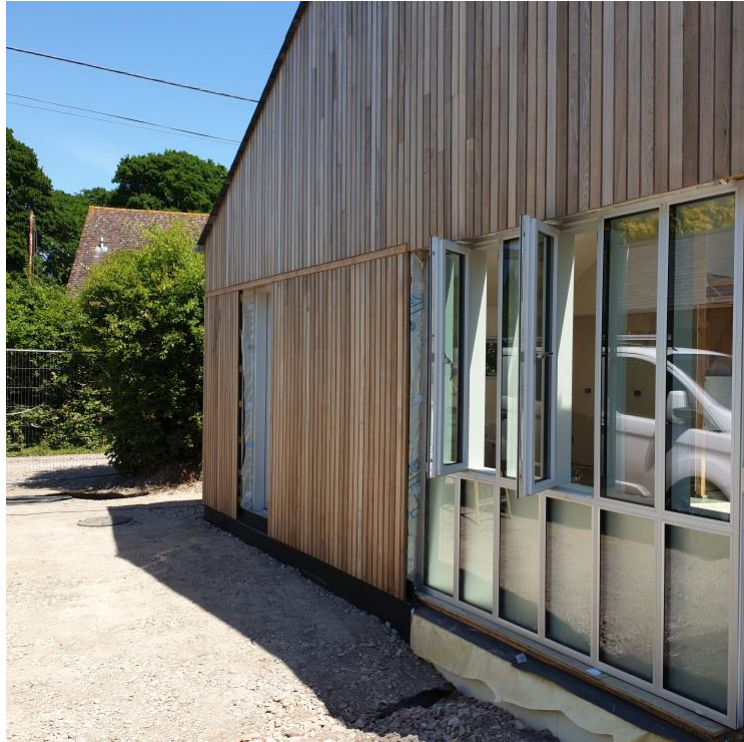
Fig. 04 (above) Construction photograph of Oakdene, Norleywood and the Ash vertical cladding.
