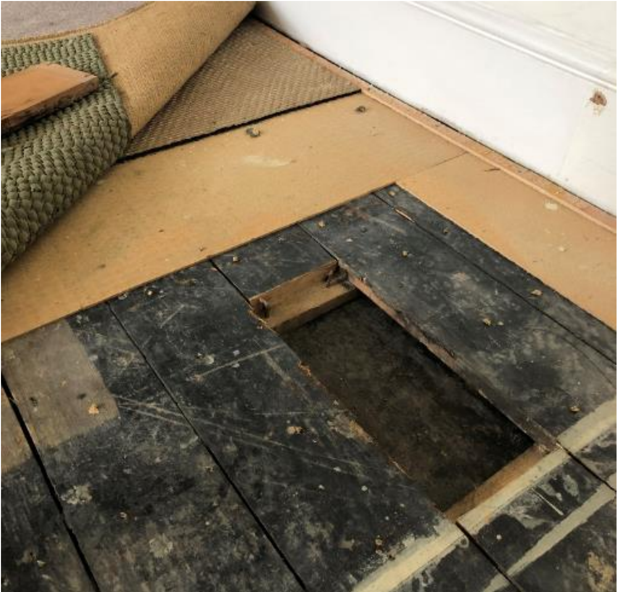
Figure 18 – Typical floor construction.
