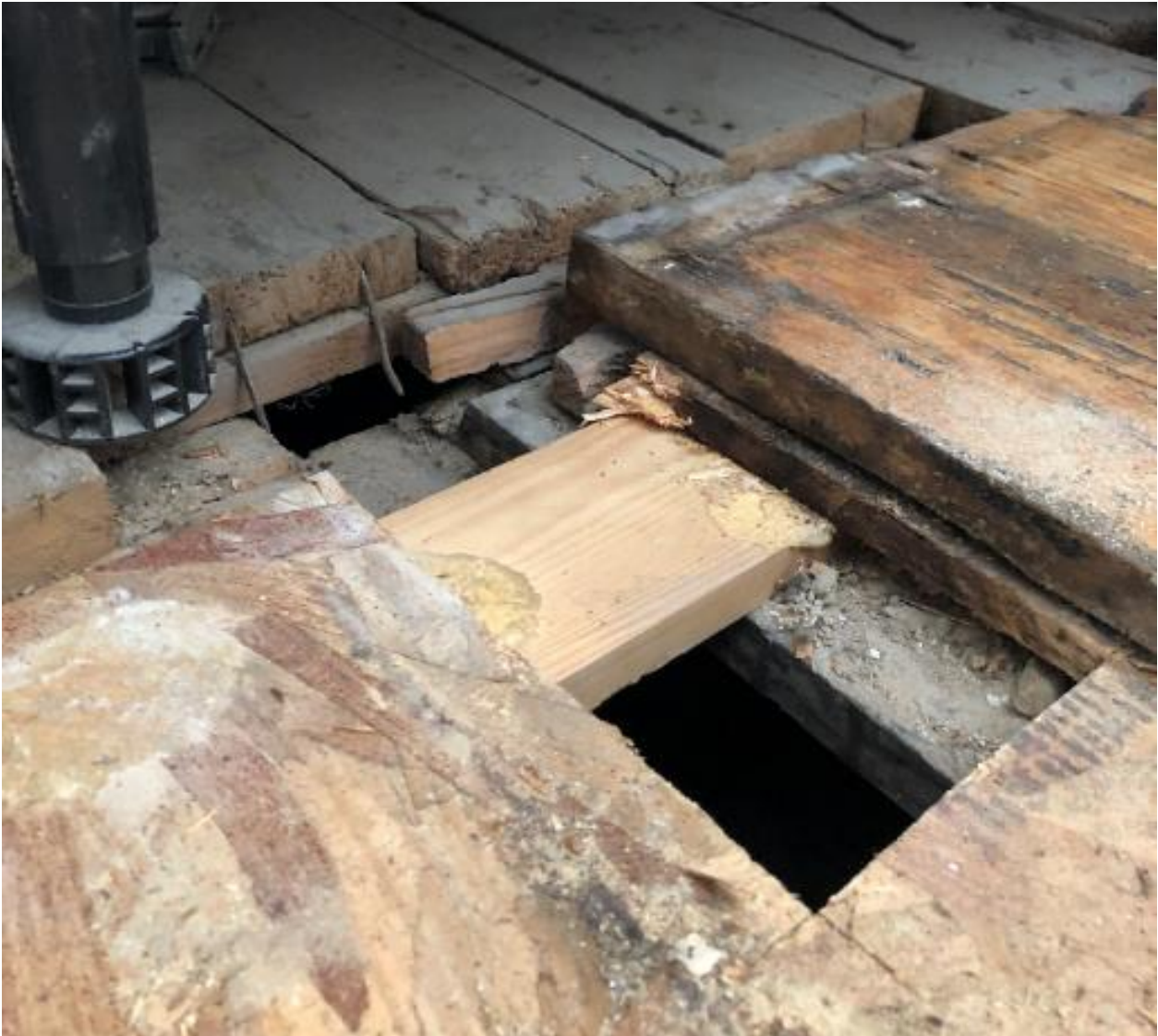
Figure 19 – Typical floor construction, kitchen.
