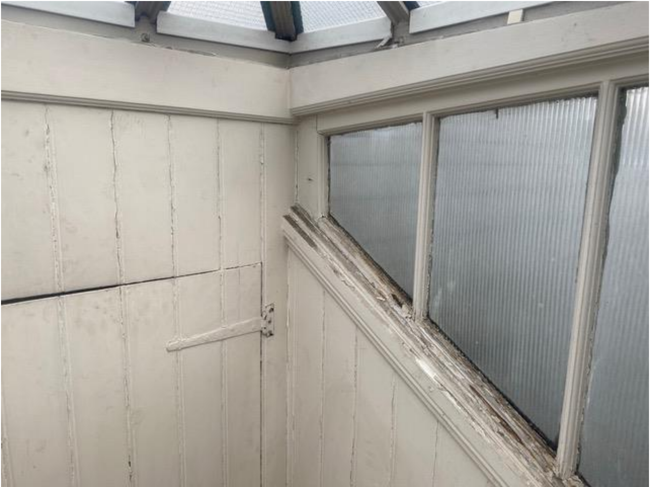
Figure 5 - The interior of the existing roof lantern.
