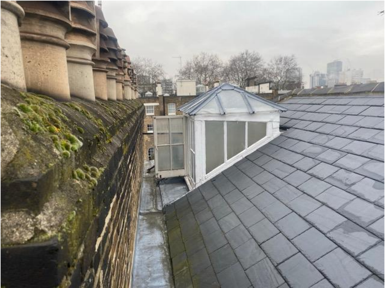
Figure 3 - The existing roof lantern, of early 20 th century construction.
