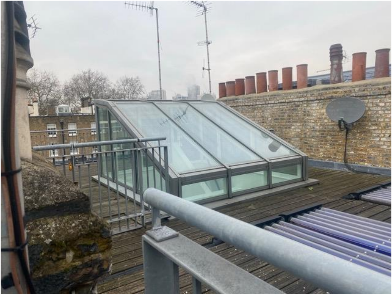
Figure 8 - Modern roof lantern (c.2008), 39 Montagu Square.
