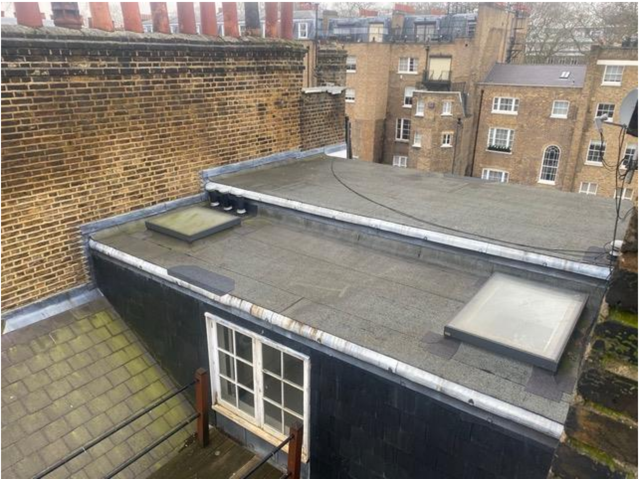
Figure 7 - Modern roof structure looking down on 41 Montagu Square.
