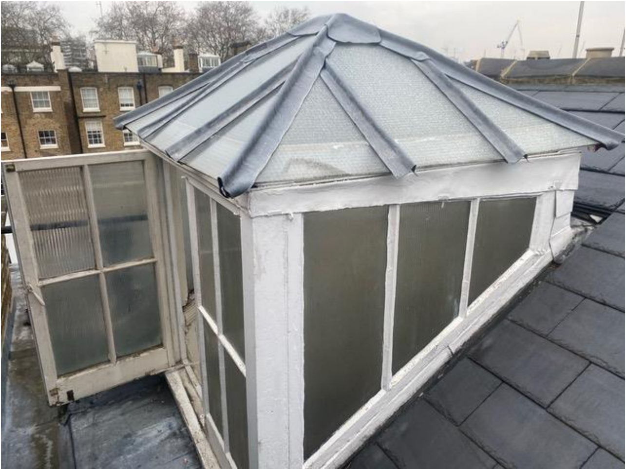
Figure 4 - The existing roof lantern, of early 20 th century construction.
