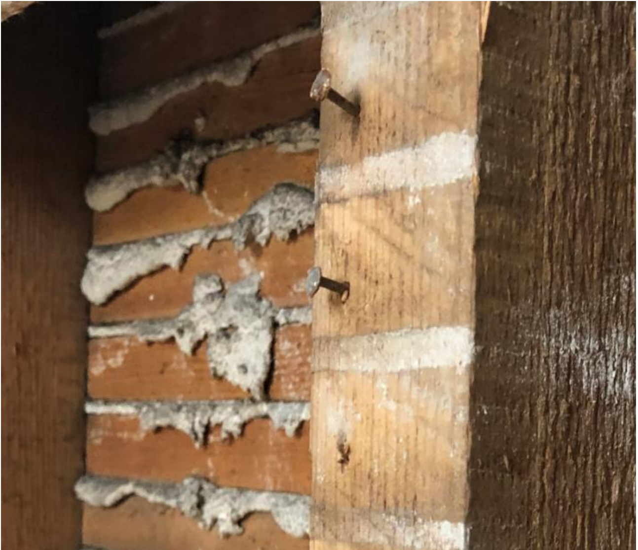
Figure 17 - Victorian-era machine made nails used to apply laths, third floor.
