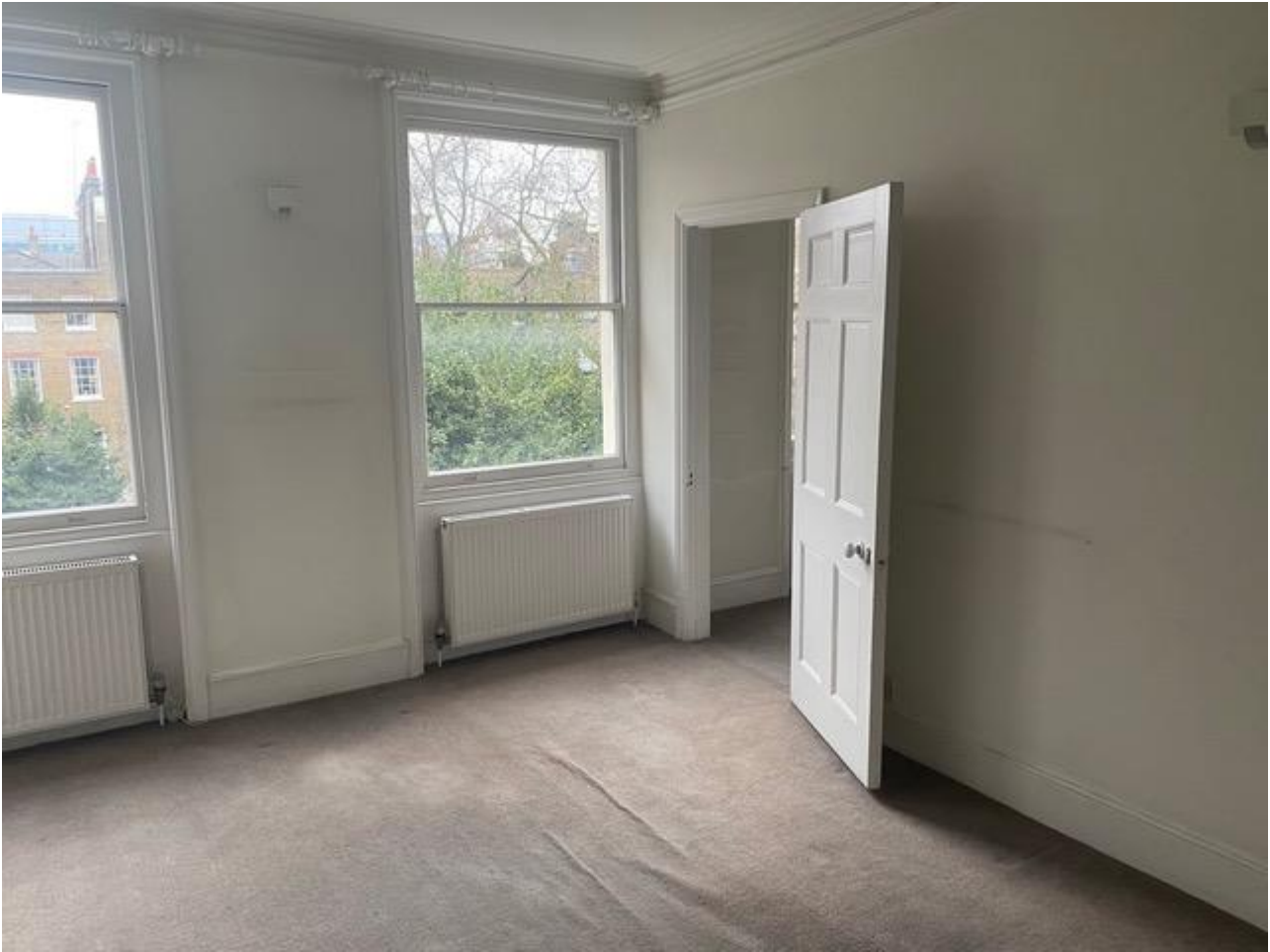
Figure 16 - Dividing wall between the large and small front room, third floor.
