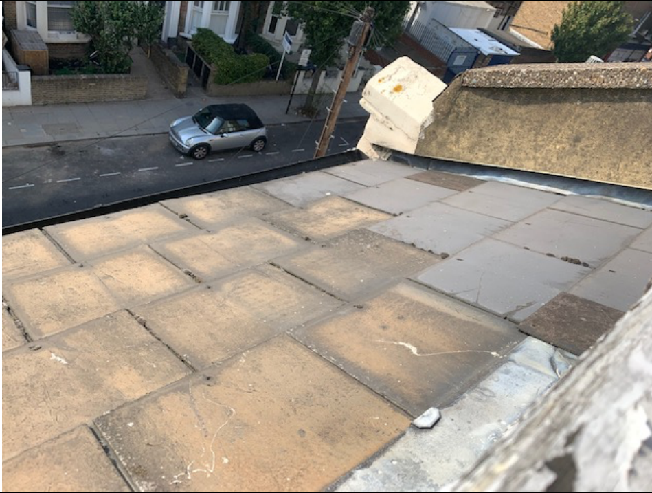
5. Pitched roofs are covered with artificial slates with hook fixings.
