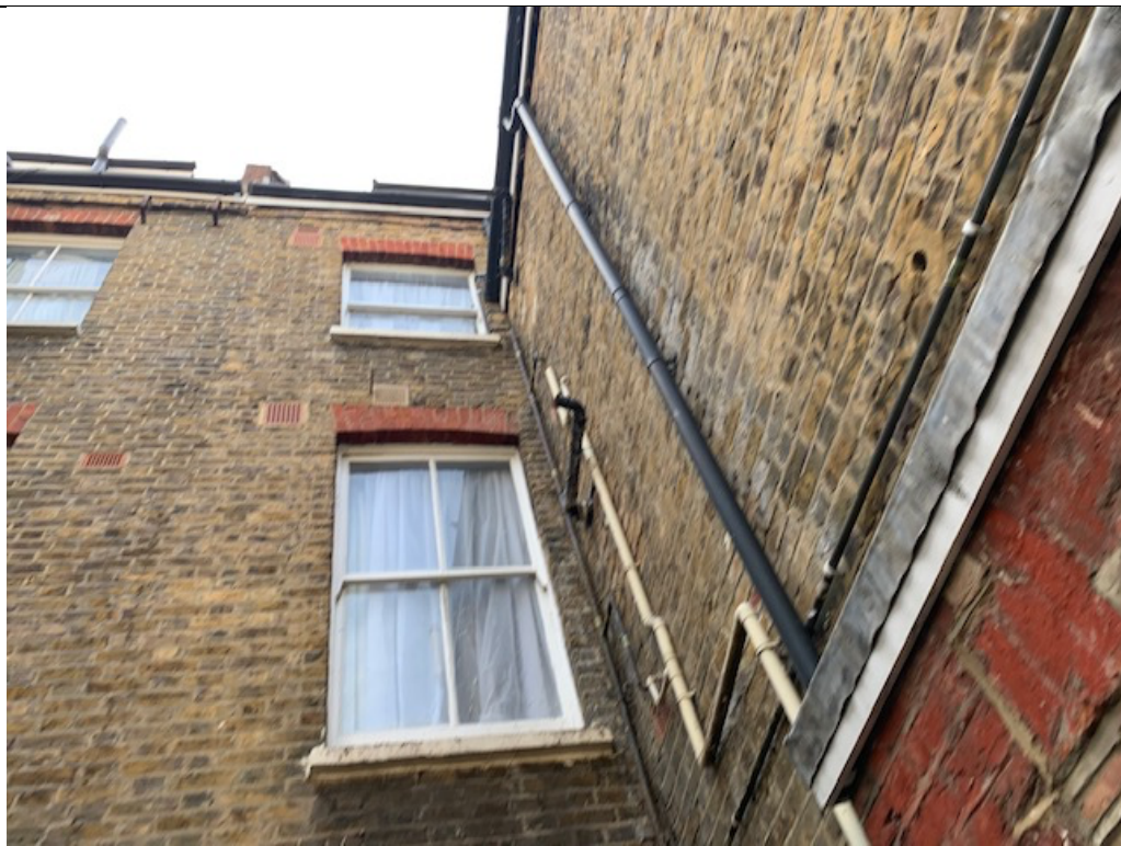
10. Close-up of rear elevation showing sash windows.
