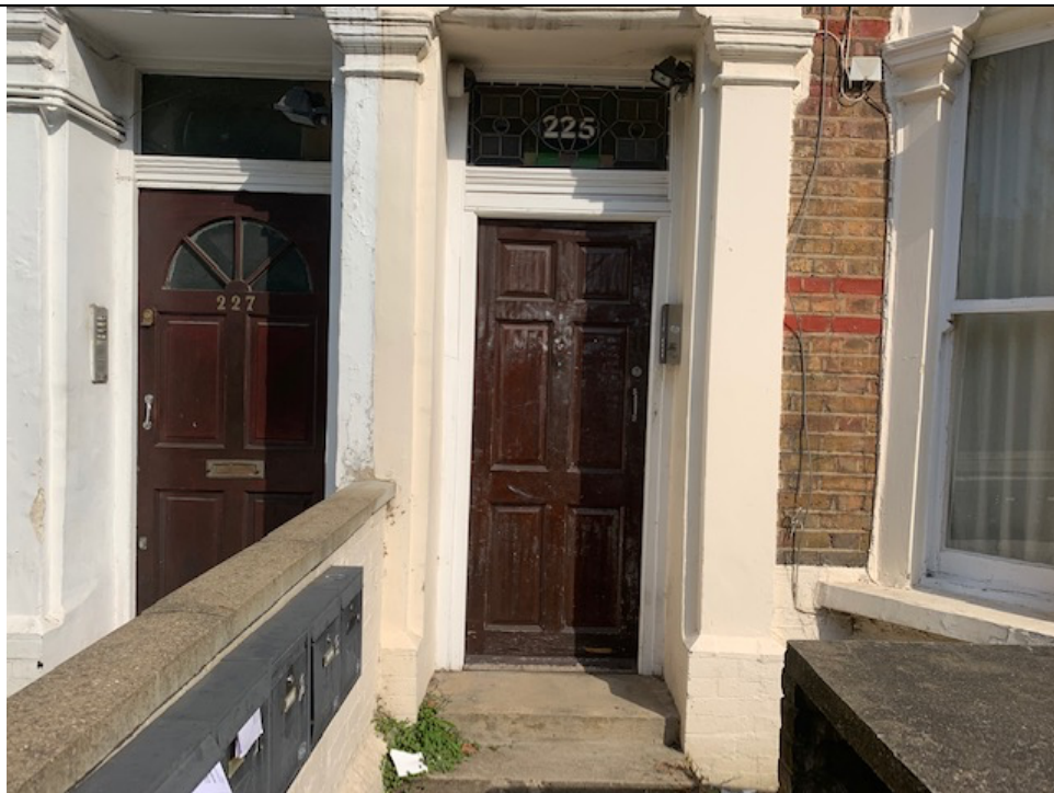
4. Front door is a traditional 6-panel solid timber door with a stained glass fanlight above.
