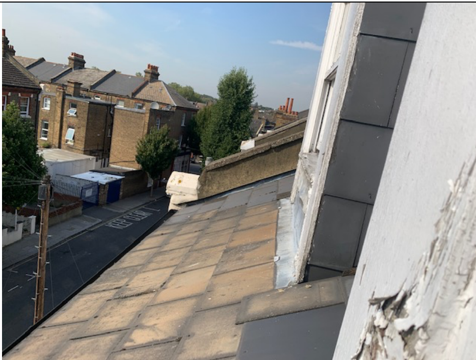
6. Dormers also have artificial slates to their cheeks (sides).
