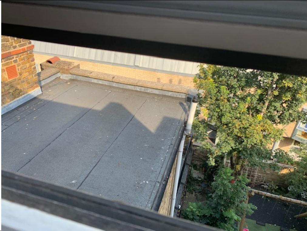
7. Rear wing/extensions have flat roofs and felt coverings.
