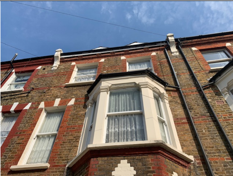
2. Close-up of front elevation showing bay window and timber sash window detailing.
