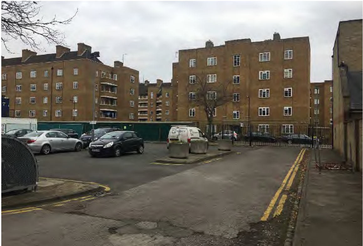
Photograph 3: Car park interior looking northeast
