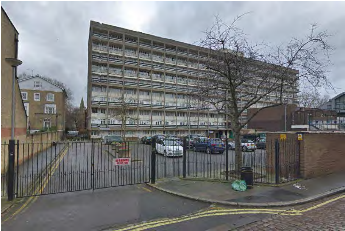
Photograph 1: Torridon House car park looking west
