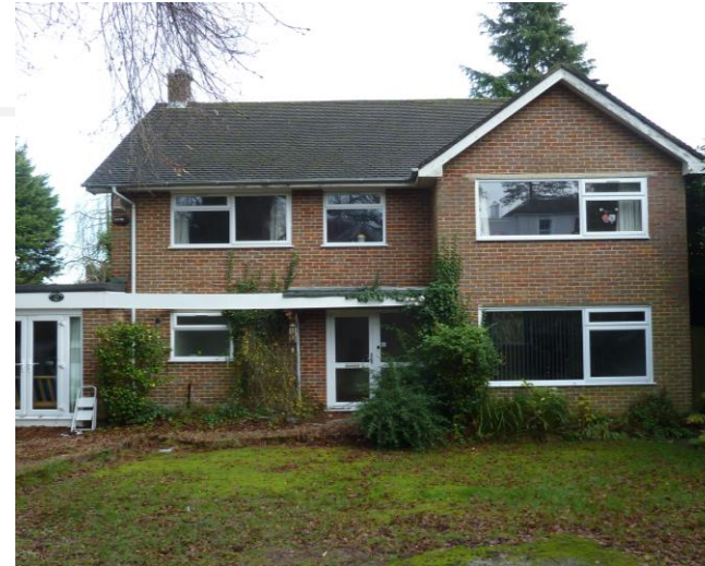
Front elevation of current property
