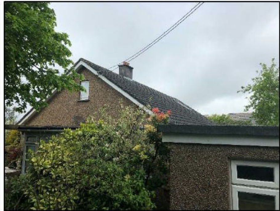
Figure 5 Rear with flat roof garage
