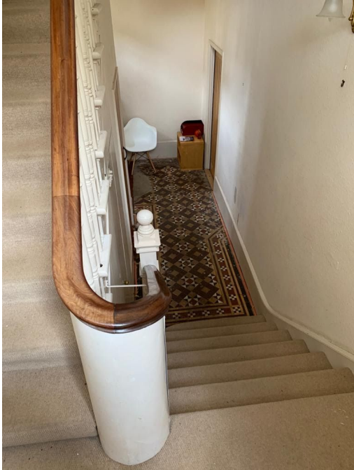
Fig 5 - View of ground floor flat door immediately below the proposed location of the first floor relocated door.
