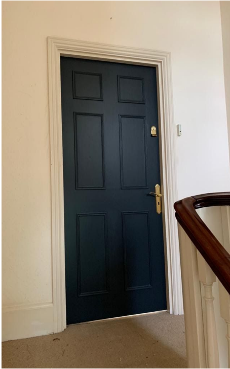
Fig 1 - Front door for First Floor Flat, 21 Downleaze (Both the wall and doorway are a non-original feature).
