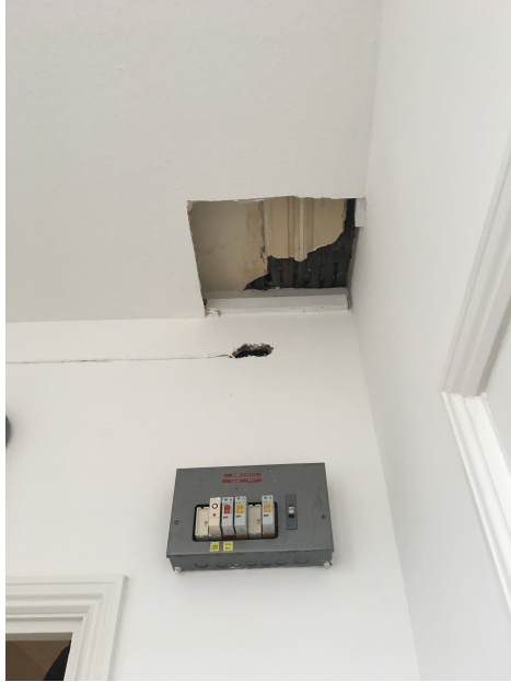
Fig 7 - False ceiling covering up original coving that was added in the 1970s conversion within the internal hallway. Proposed plans will not impact on the corincing.
