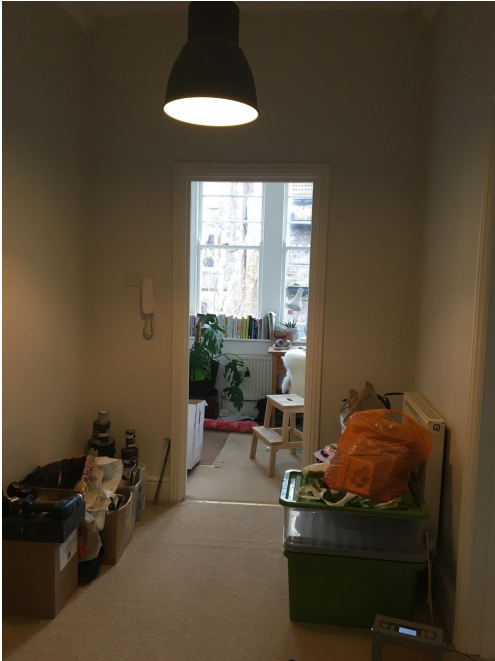
Fig 6 - Internal hallway of First Floor Flat showing non-original stud wall at end of hall.
