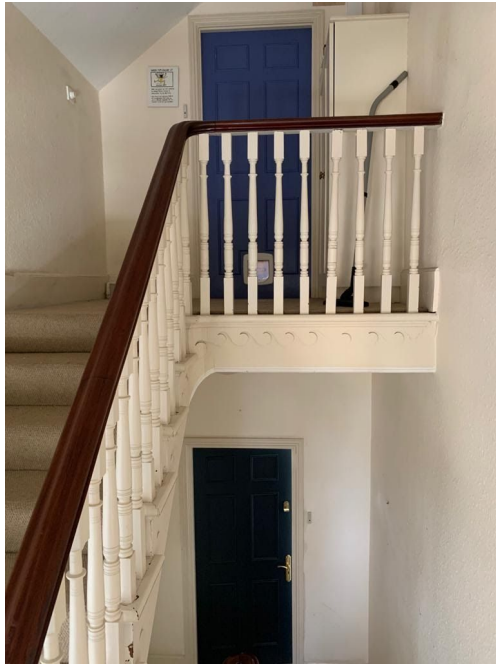
Fig 3 and 4 - Front doorways for top floor flat and ground floor flat (both doorways are a non original feature and were added in the 1970s conversion).
