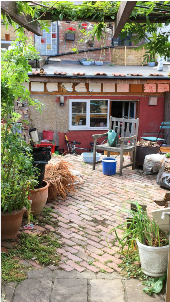
1. Rear Elevation view including rear garden with higher ground level and single storey area.
