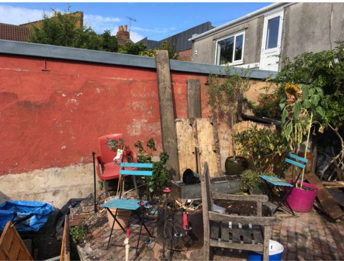
3. Rear garden with higher ground level. Boundary with no. 300 North Street and extension within no.300 running continually along boundary.
