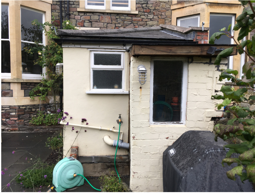
3. Rear Elevation view of existing extension
