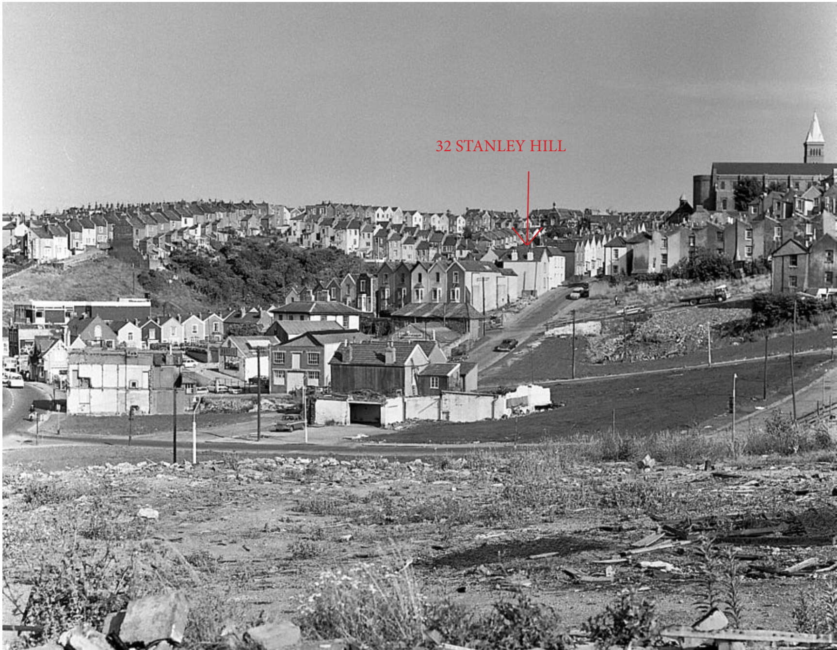
Photo of the site after demolition.
