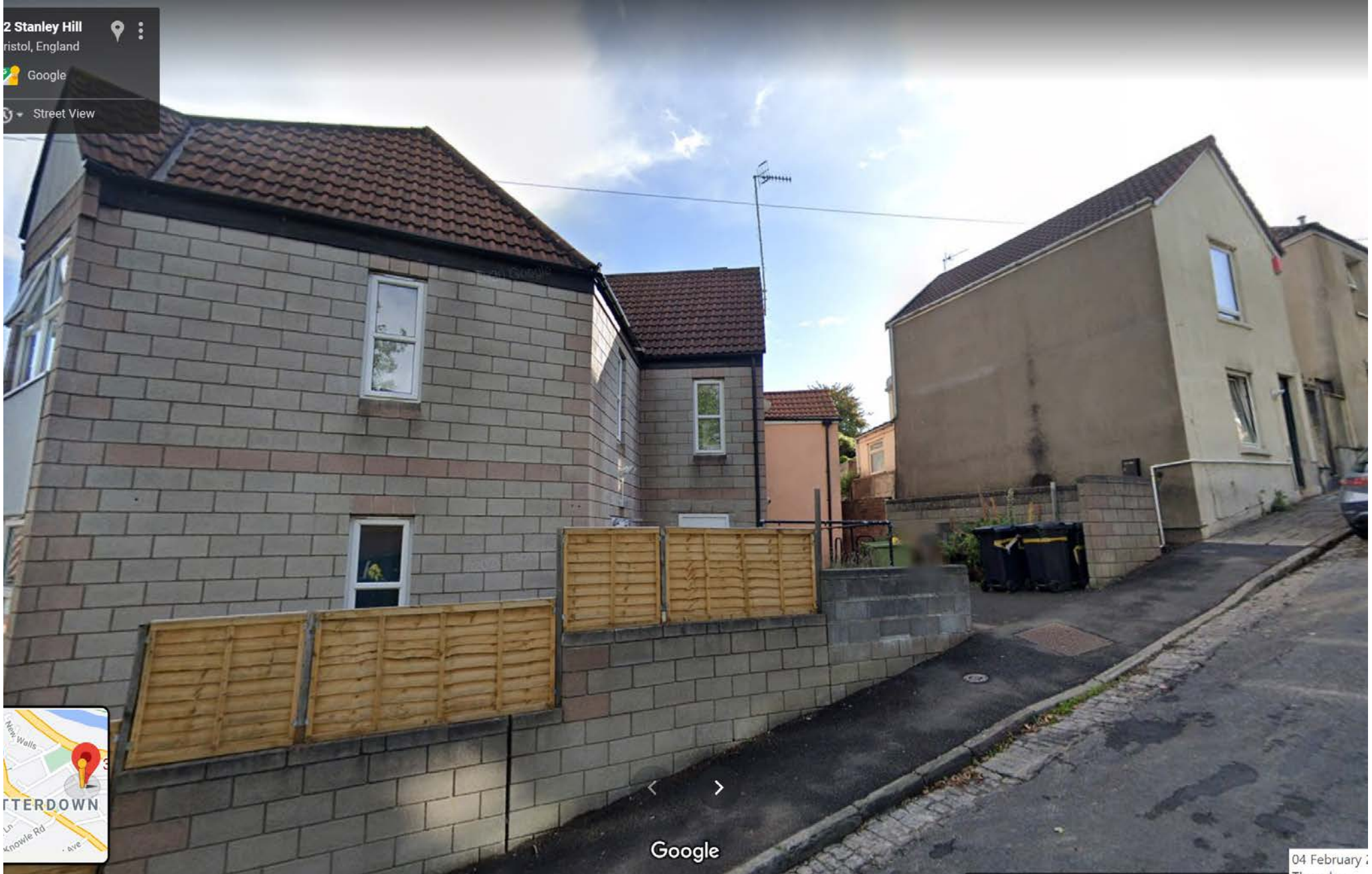
View of St.Mungus Centre and Side elevation 32 Stanley Hill.
