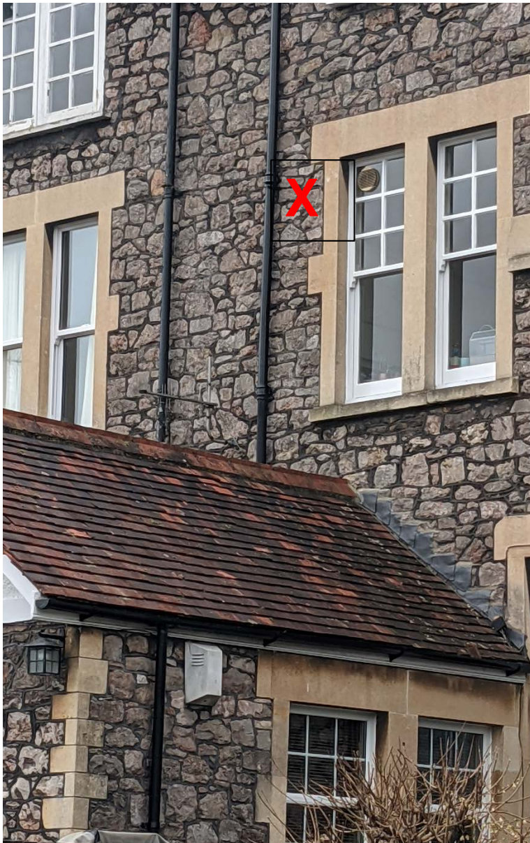
Photograph: Outside of the building (rear)
